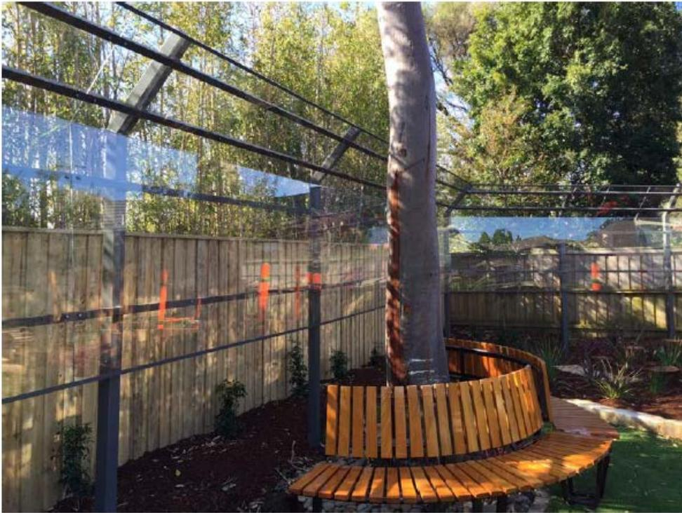
**Figure 3: Representative image of acoustic barrier**
