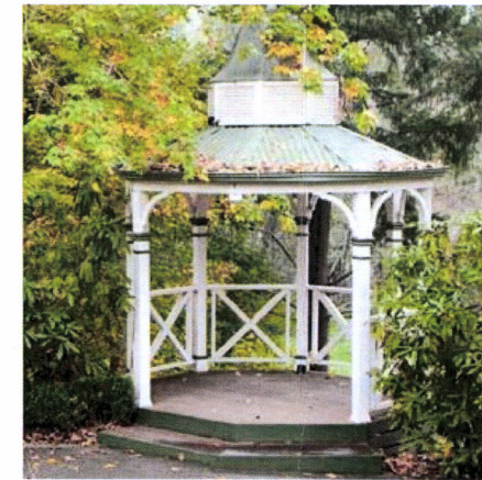
Pavillion / Gazebo Structure
