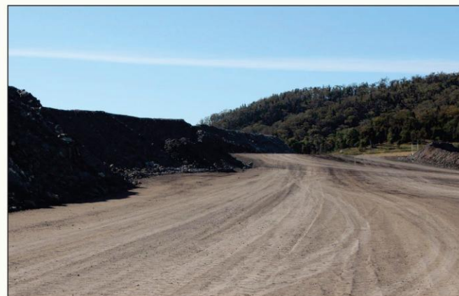
Plate 4 Typical berms/bunding along haul roads
