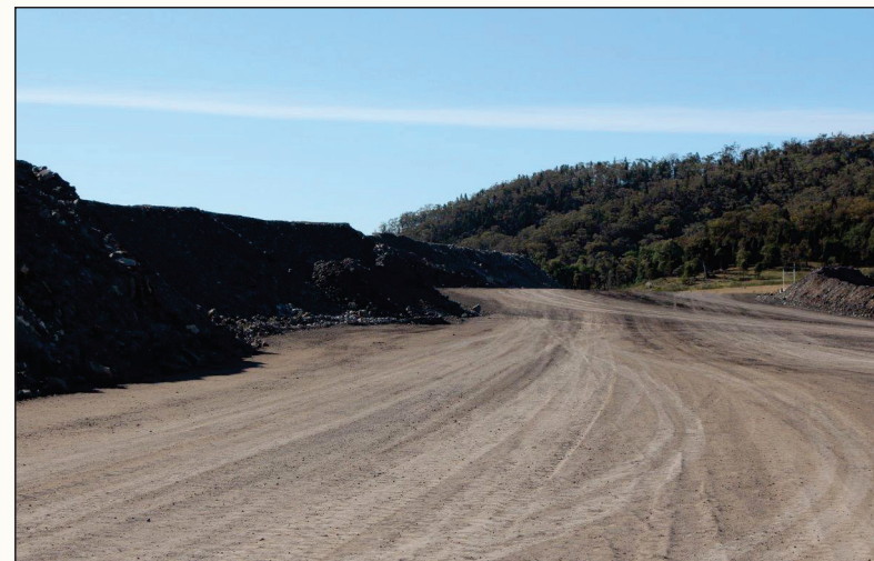
Plate 4 Typical berms/bunding along haul roads
