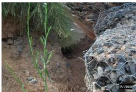
**Fig1.5** River bank erosion adjacent to the gabion at the outlet in Lawson ark.
