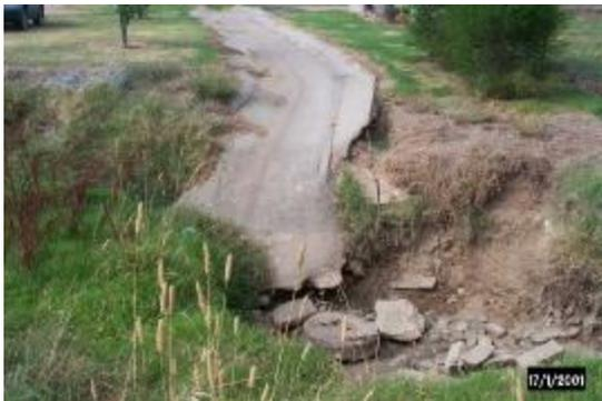
**Photo 3.** Erosion and debris around the street drainage outlet at the end of Court St, Mudgee
