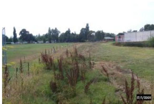
**Fig1.4** The grass swale adjacent to the constructed wetland
