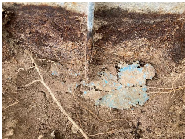
Figure 8 – Waterproof membrane
