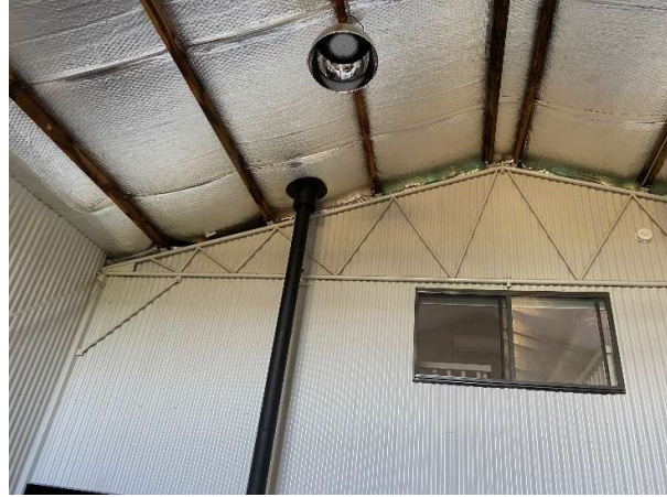
Figure 6 – Fully clad end bay
