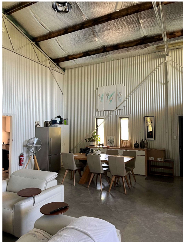
Figure 4 – Internal roof trusses and bracing
