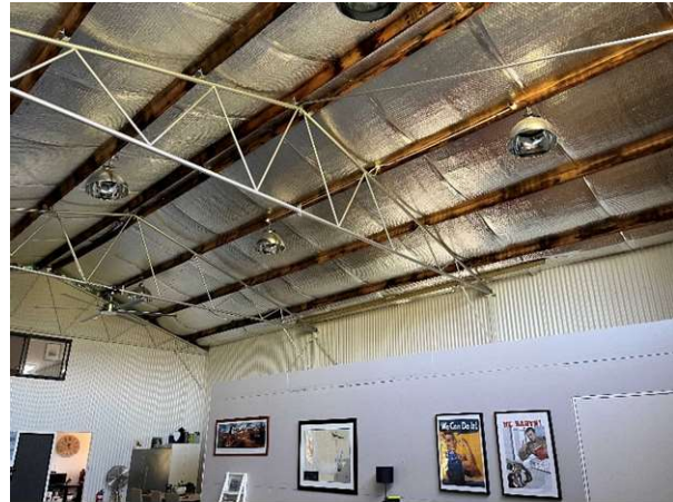
Figure 2 – Internal roof trusses and bracing
