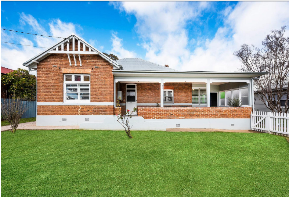
2 PHOTO - NORTH FACADE BEHIND FENCING
