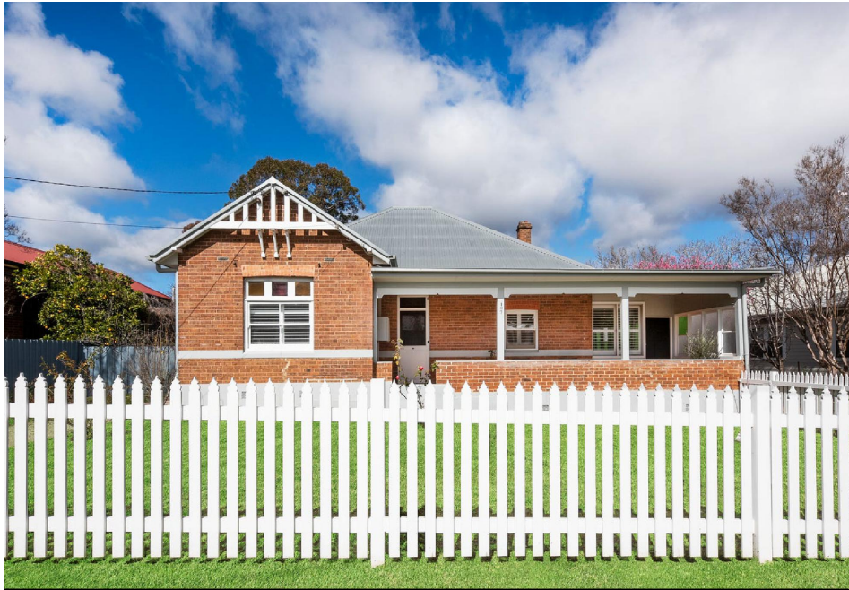
1 PHOTO - NORTH FACADE FROM FOOTPATH SHOWING FENCING
