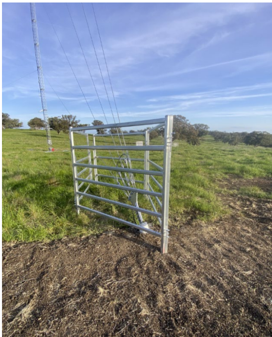
Figure 7: Example of finished buried anchor, post construction – with cattle fencing
