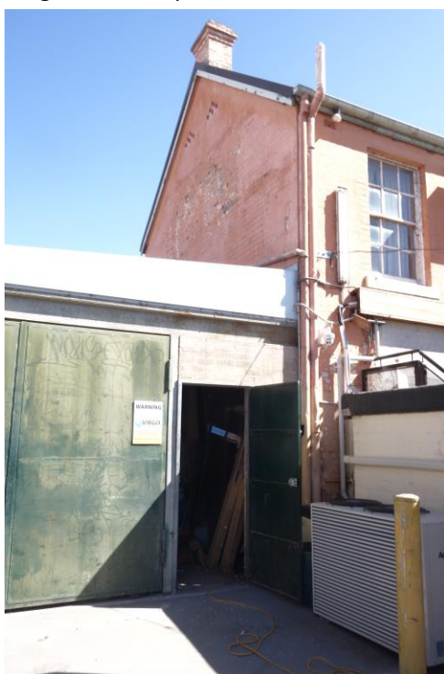
Figure 6 Original timber framed double hung window, 6 lights per pane to be repaired and conserved. Figure 7 Visually intrusive services to be relocated.
