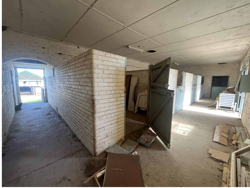
6. REMOVE NON-ORIGINAL BRICK STALLS & CEILING
