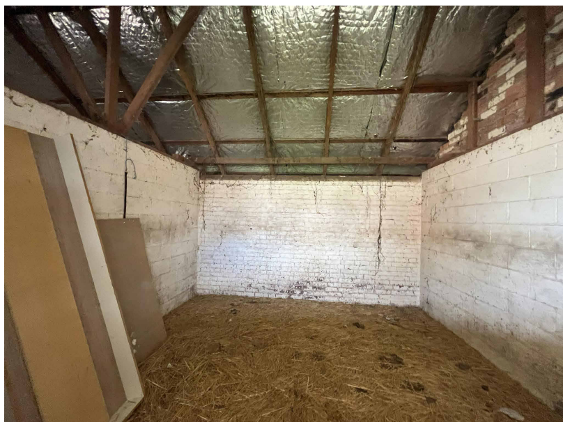
2. REMOVE WALLS & ROOF, RETAIN ORIGINAL BRICK WALL
