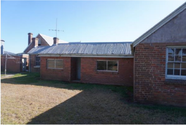
Additional Flat facing south -stretcher bond
