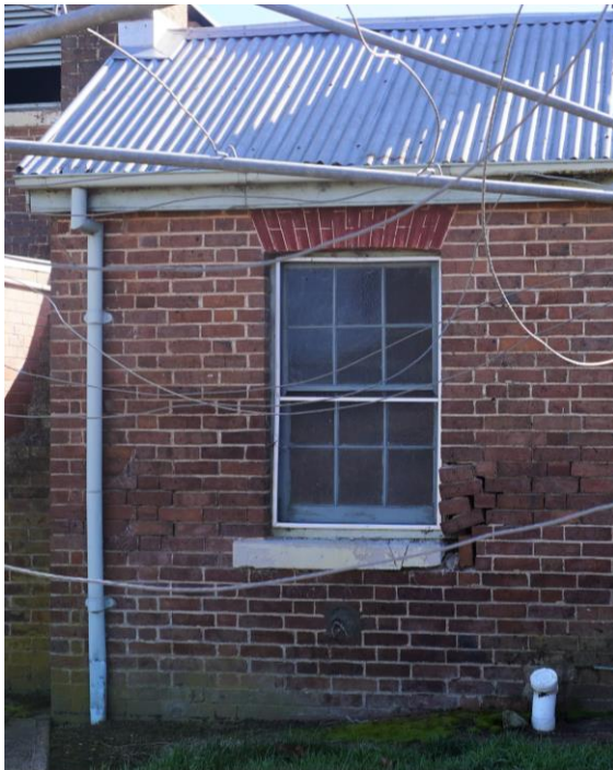
Figure 23 Shower and toilet installed in west room wing showing collapse of wall above the wc cistern.
