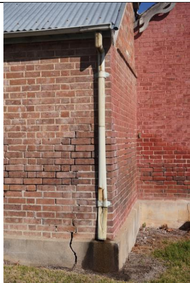
Down pipe unconnected, ground settlement crack.
