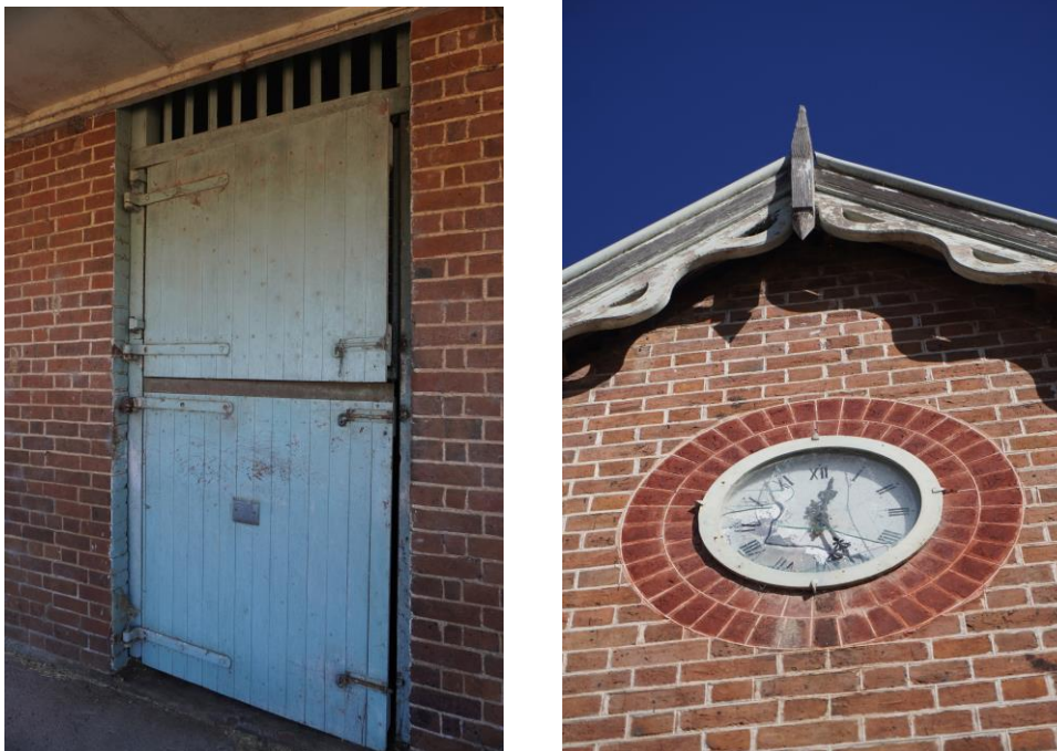
Figure 22 : Original solid timber stable doors with ventilation over; central courtyard clock mounted in the decorative gable and Flemish bond brickwork with hooks to accommodate espalier plants.
