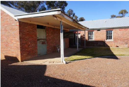
Stables added behind front wall- stretcher bond.
