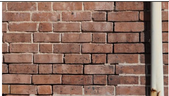
Wall detail – eroded mortar
