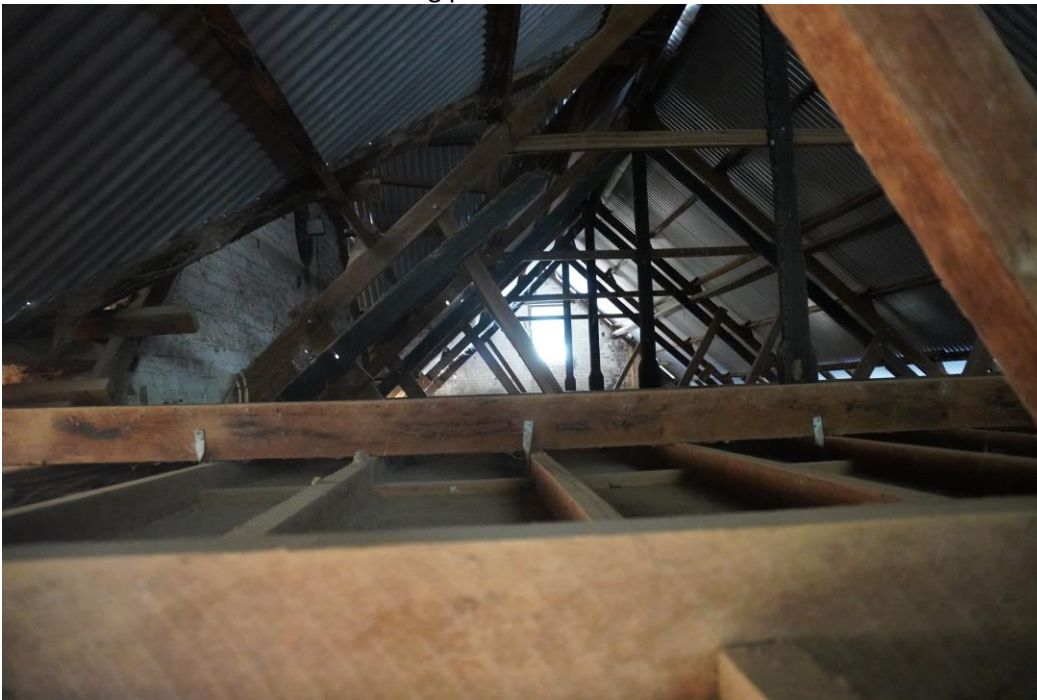
Figure 8 South end of roof space showing charred roof members.
