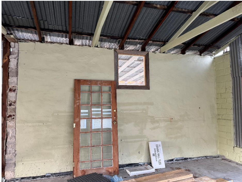
Figure 11: Block wall to be replaced with double brick
