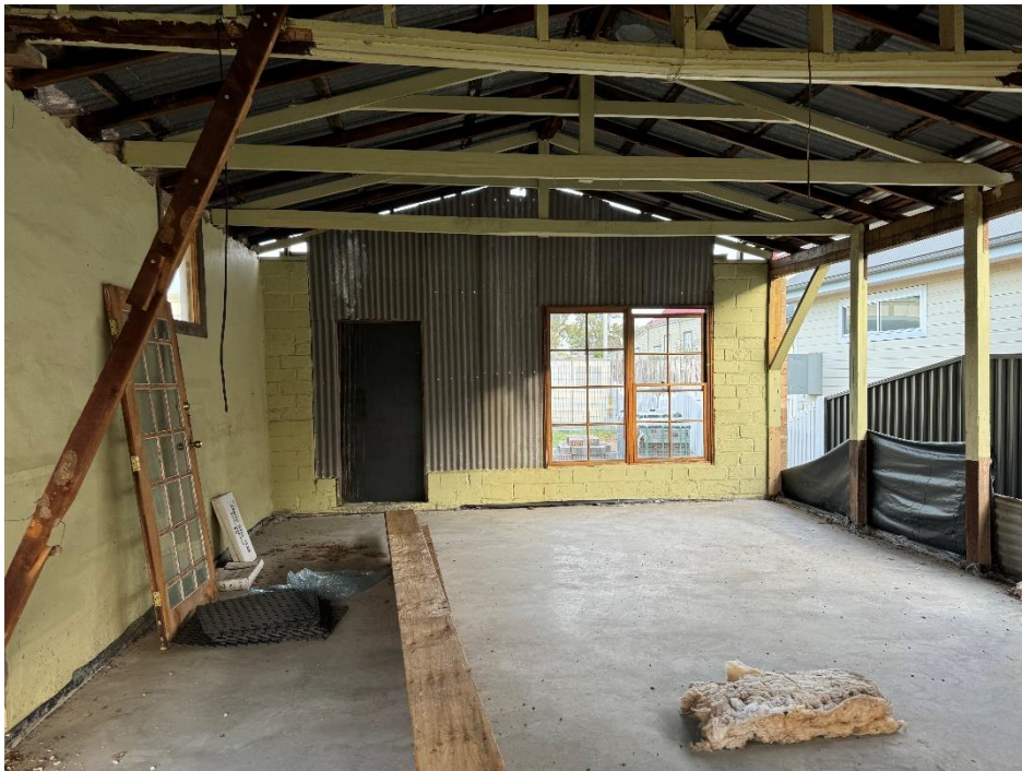
Figure 8: interior of South section, block walls to be replaced, roof framing to be supported on double brick walls
