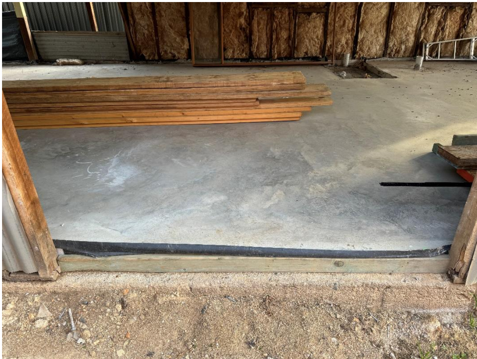
Figure 4: New 100mm topping slab with plastic membrane installed over original slab
