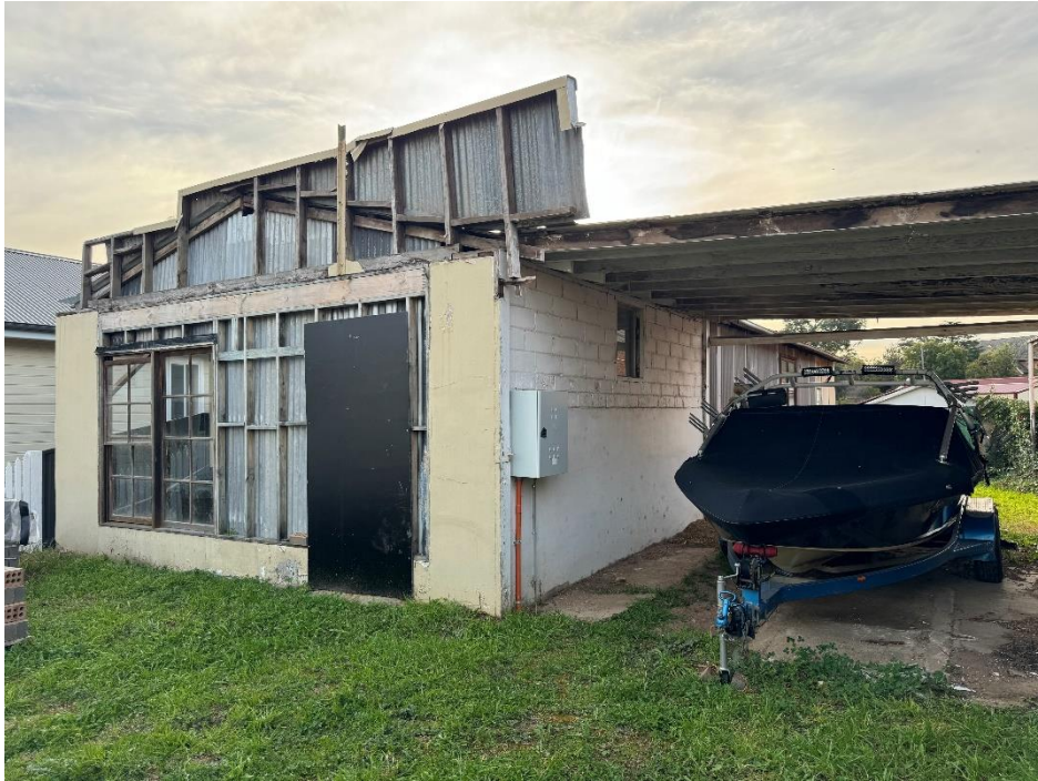
Figure 1: South elevation, block walls to be replaced with double brick, timber framing to be removed
