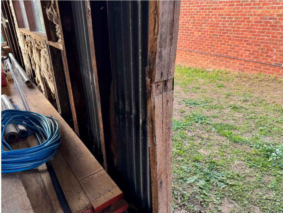
Figure 5: Damaged timber stud requiring repair as part of renovations
