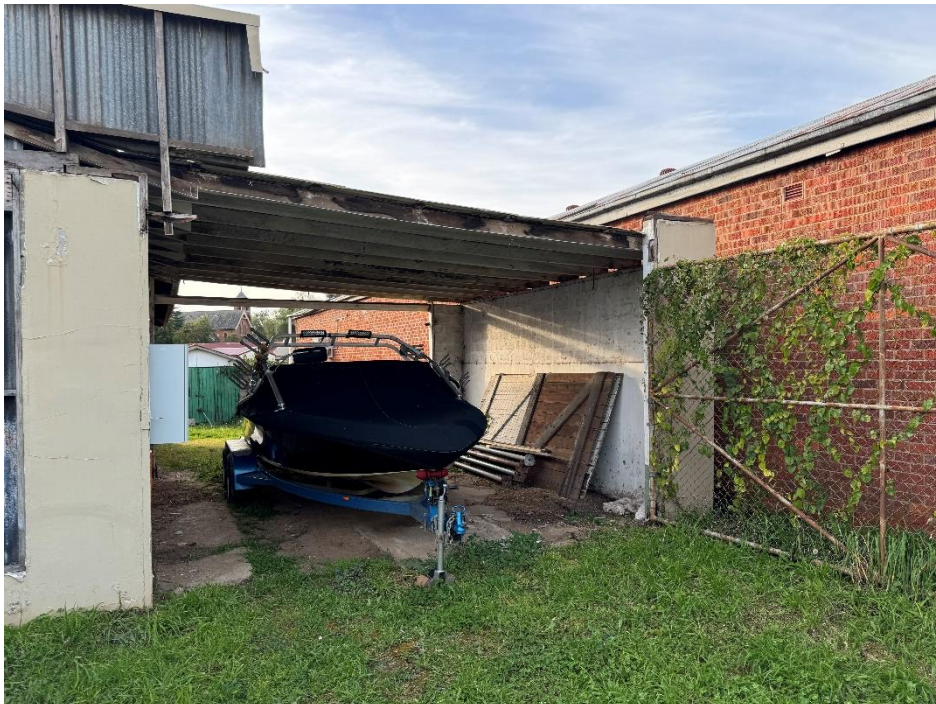
Figure 2: Skillion to be enclosed with double brick walls, existing wall and rafters to be replaced, new slab to be poured
