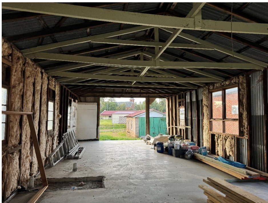
Figure 12: Existing timber roof framing generally in good condition, some repairs required
