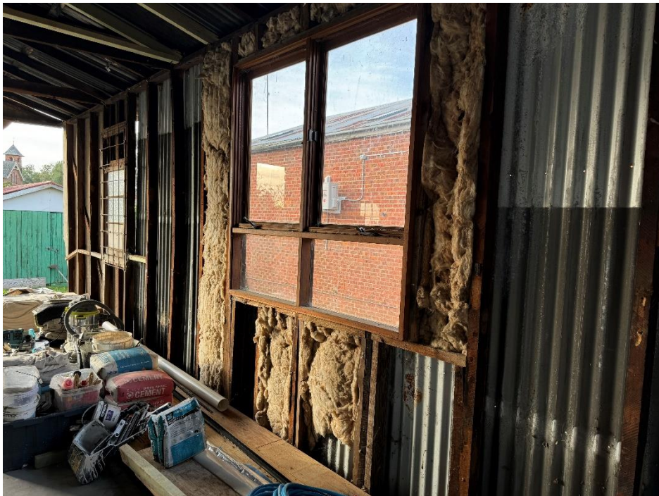
Figure 6: Hardwood wall framing generally in good condition
