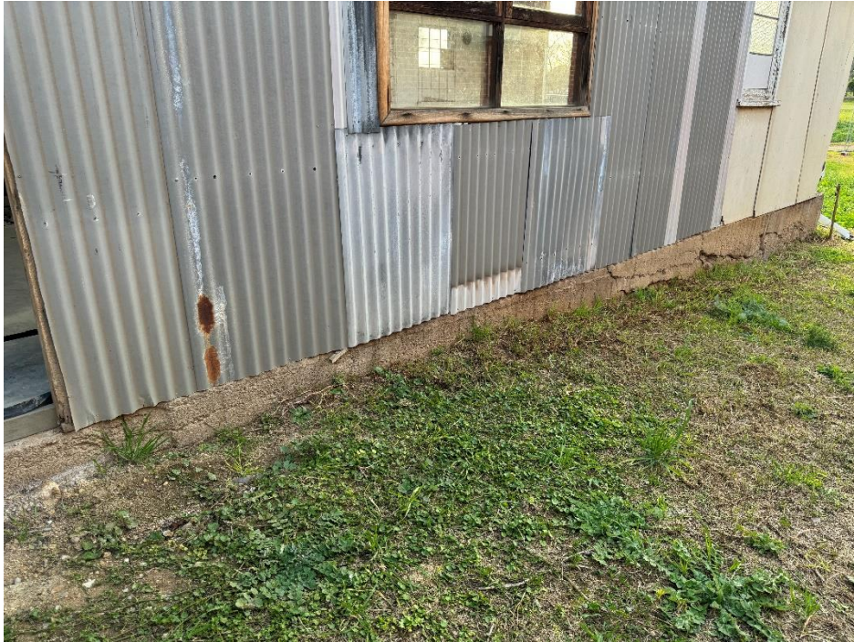
Figure 3: Existing slab, with deep edge beams due to ground slope
