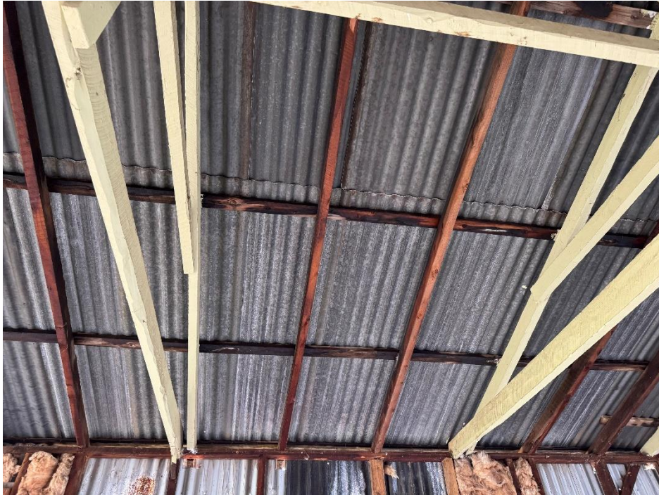
Figure 13: Existing timber roof framing generally in good condition, some repairs required, raked ceiling proposed
