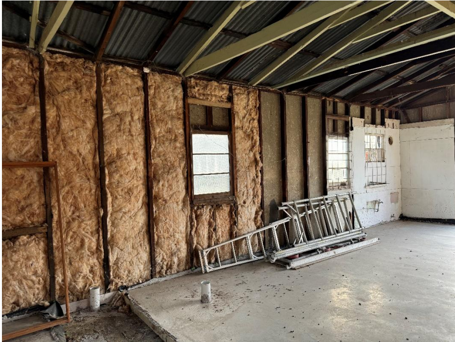
Figure 7: Hardwood wall framing generally in good condition
