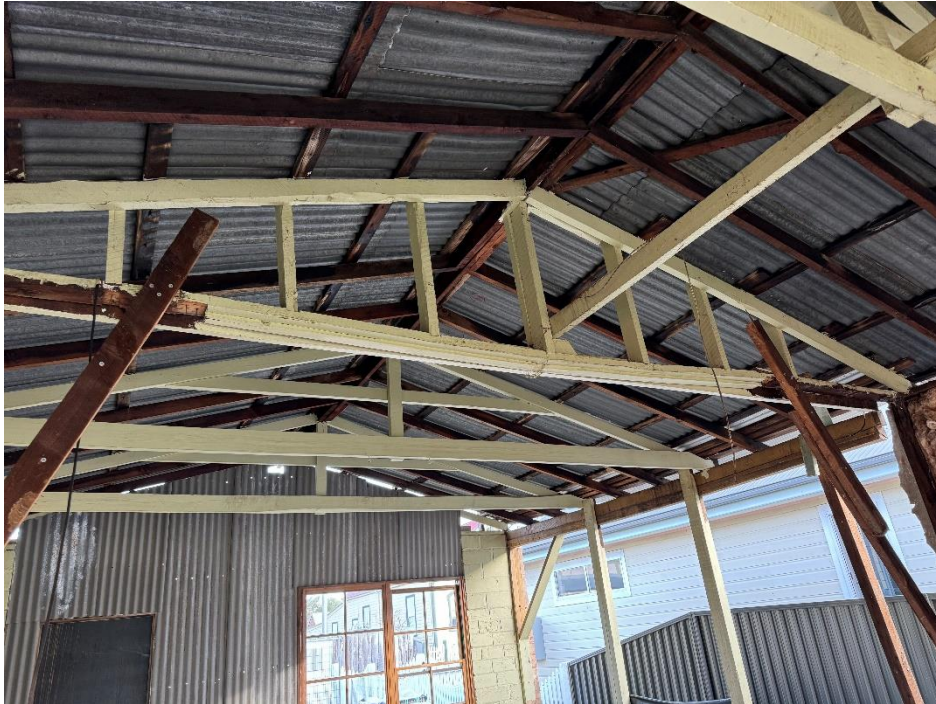
Figure 9: Existing timber roof framing, some damage noted with repairs to be provided as part of renovations
