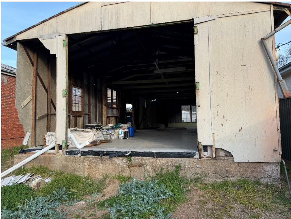
Figure 14: North elevation, cladding to be replaced
