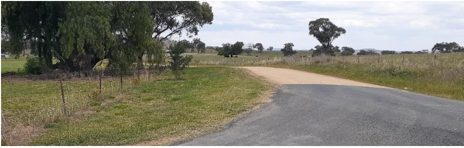
Photo 5: Zimmer Lane looking left along Grimshaw Lane
