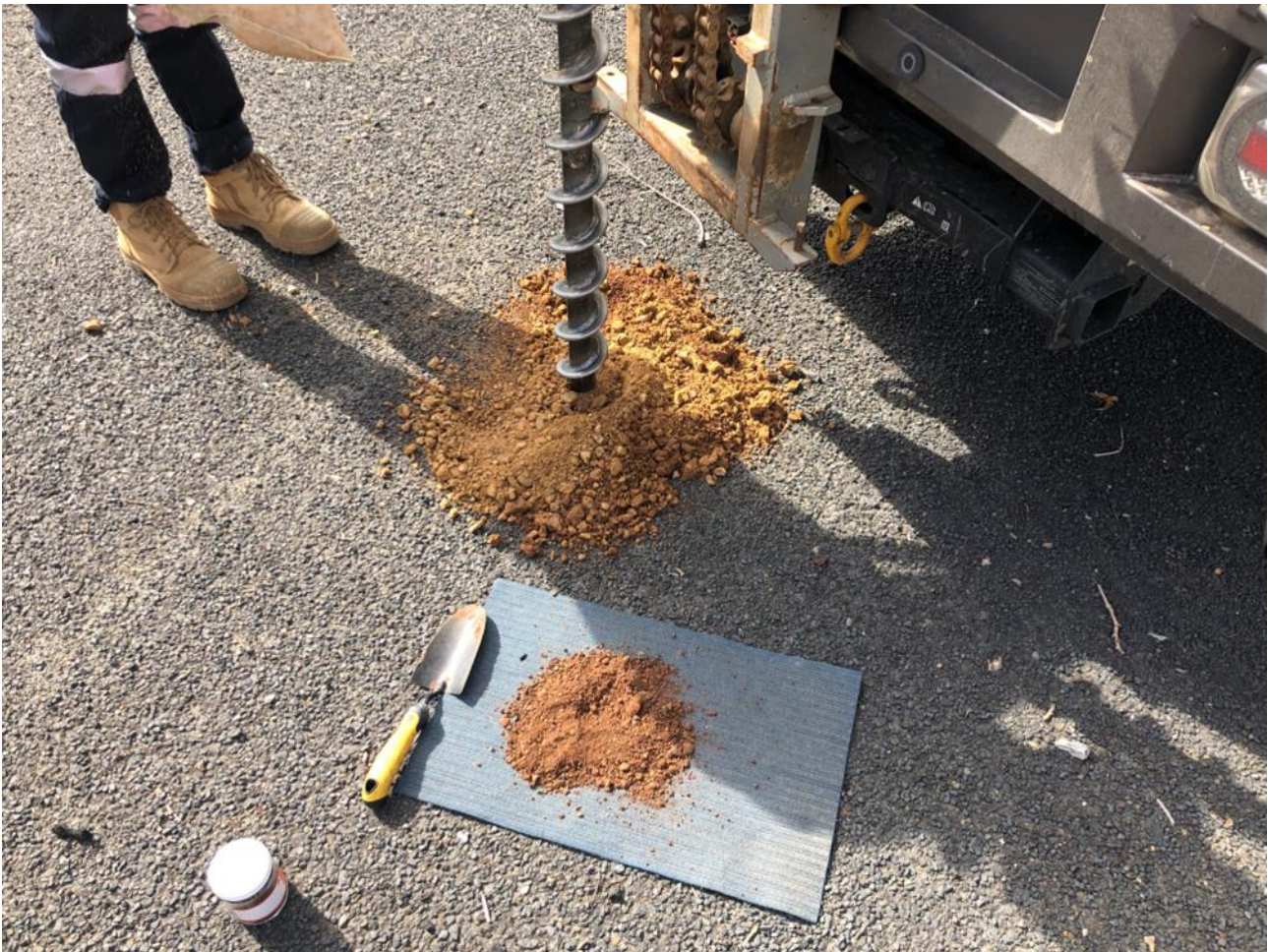
Figure 5.8: Geotechnical auger drill bore into hardstand of the former carpark.
