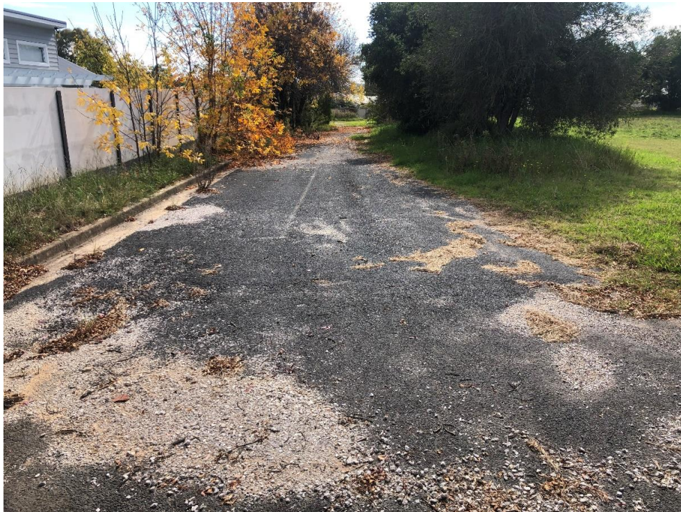
Figure 5.3: Northern driveway providing access from George Street
