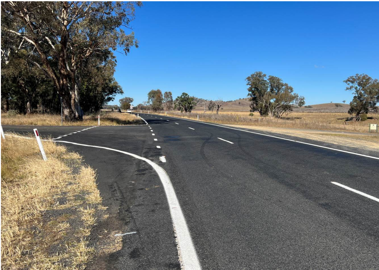
Photograph 5 – Guntawang Road near Magpie Lane.
