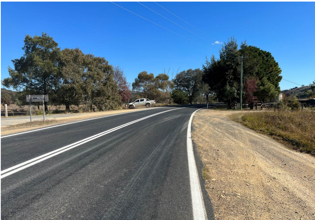
Photograph 6 – Guntawang Road near the Castlereagh Highway
