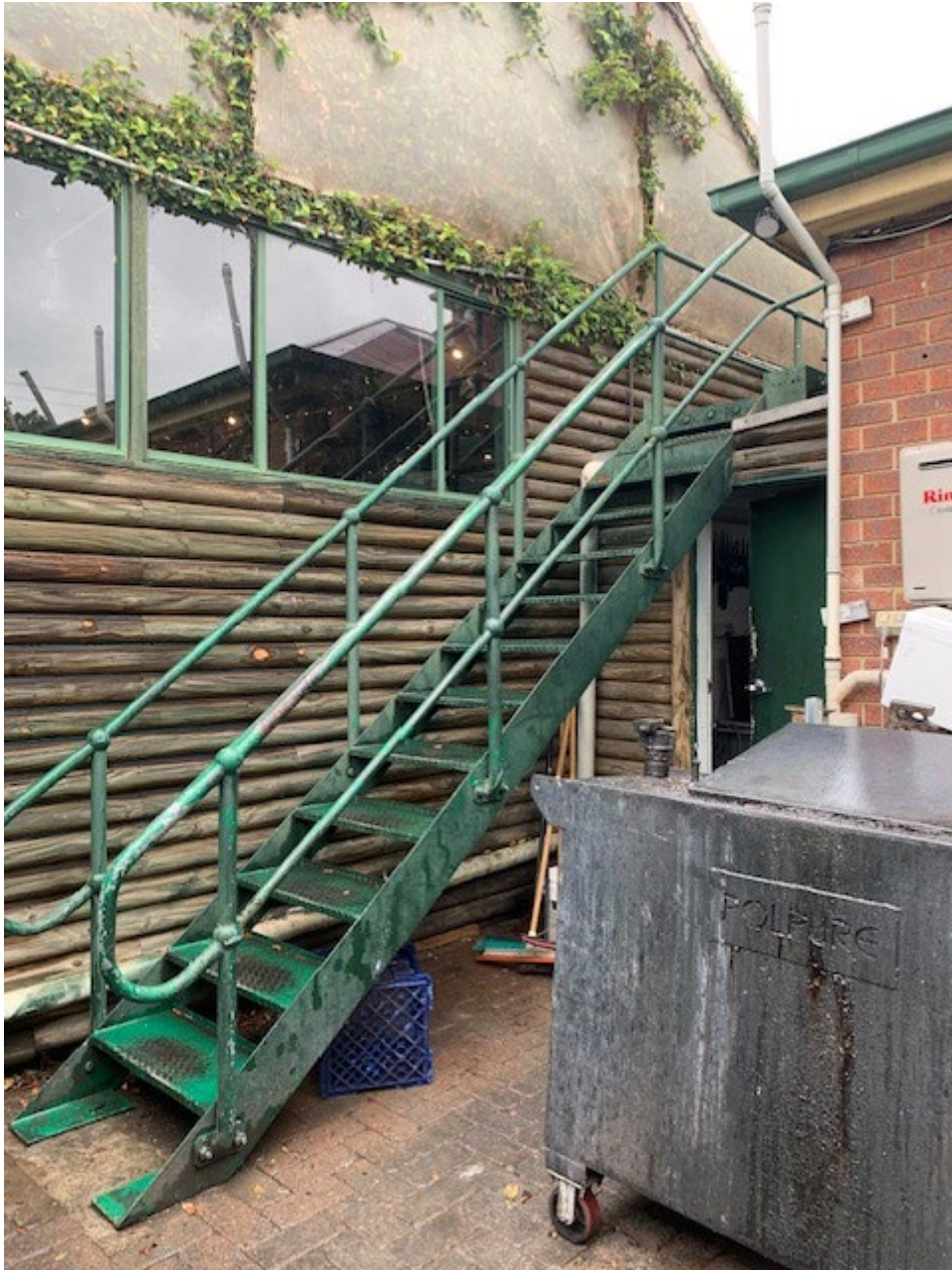
Image 02 Existing Metal Stair
