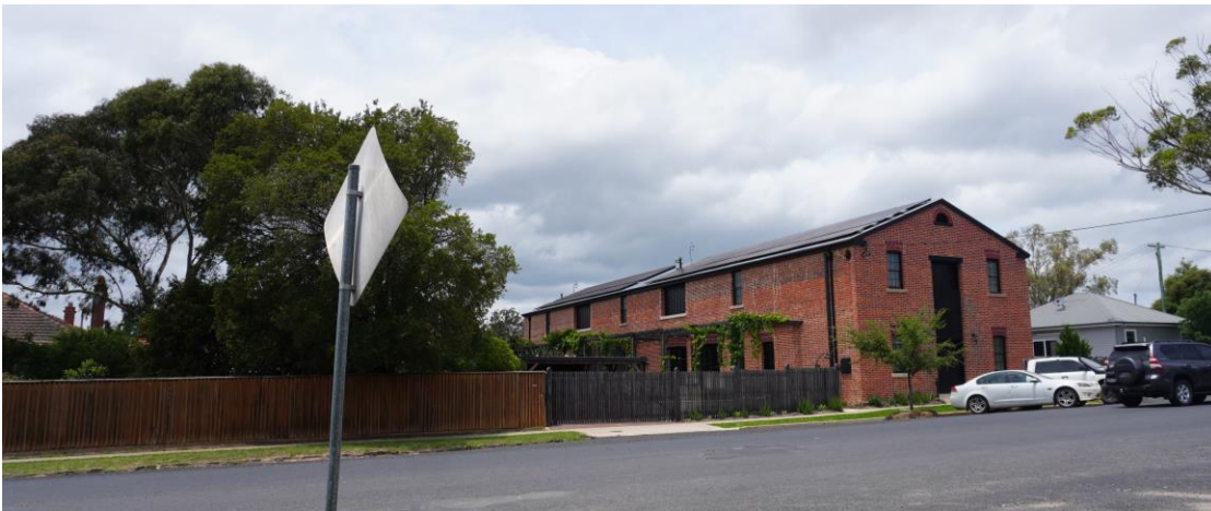
Figure 1 The Lewis Street Former Warehouse façade. 15 Jan 2024. BjH
