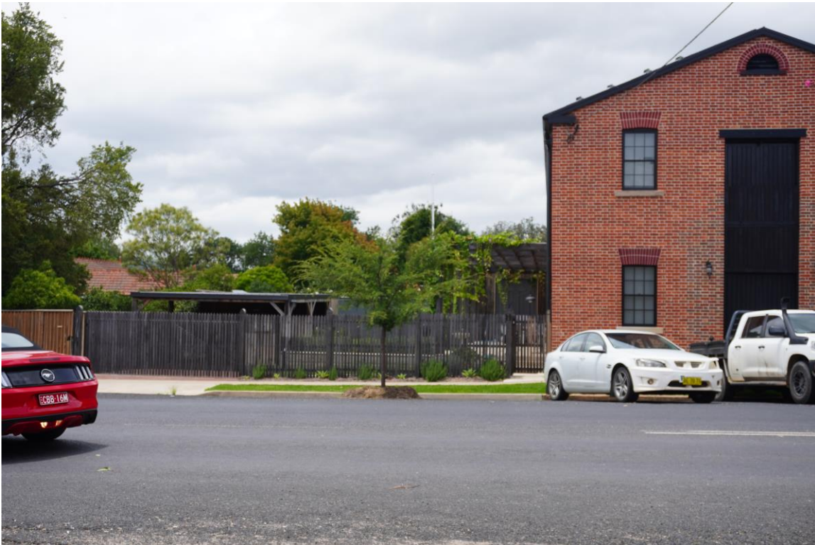
Figure 4 View of the carport and its relationship with the former Warehouse 15 January 2024
