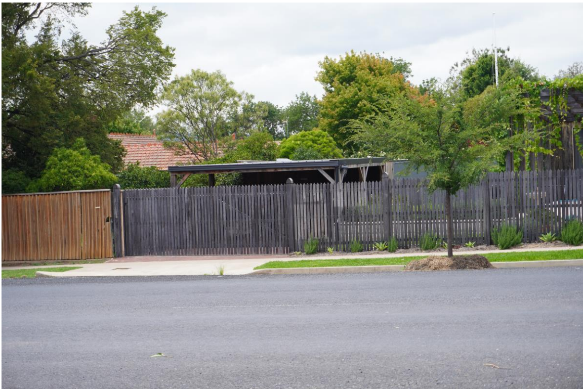
Figure 3 The Lewis Street Carport façade. 15 January 2024
