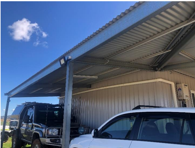
Figure 7 – Verandah attached on South-West side of converted shed
