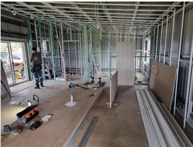
Figure 3 – Exposed timber framing of partition walls (client supplied)
