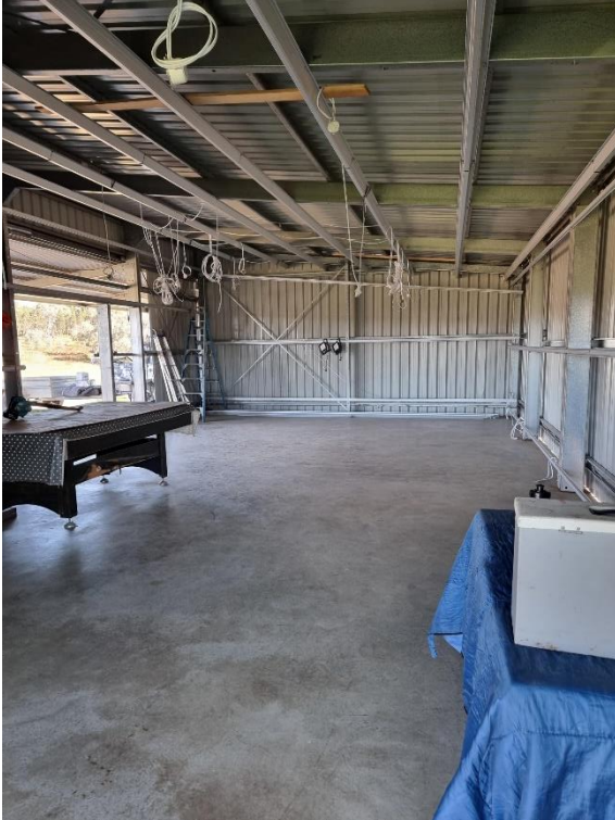
Figure 1 – Top hat battens installed to support ceiling lining (client supplied)
