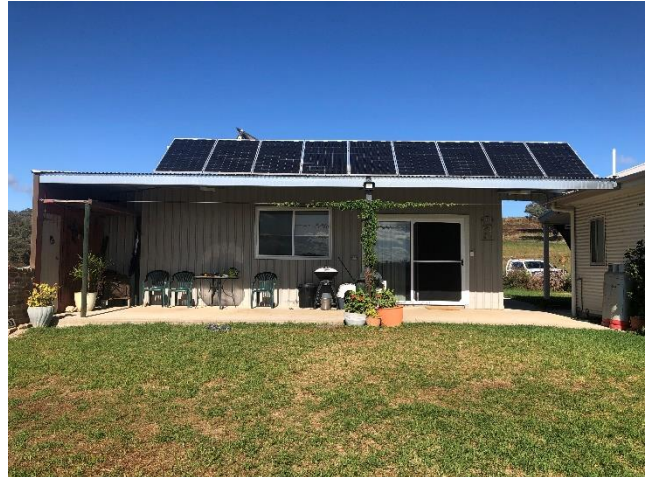
Figure 6 – North-East side of converted shed
