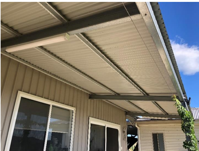
Figure 9 – Framing of attached verandah roof on North-East side of converted shed
