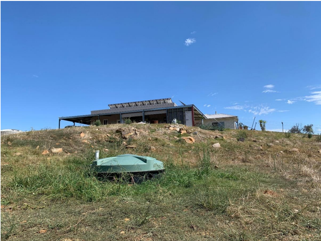
Plate 4 – Existing Plastic Septic Tank Location
