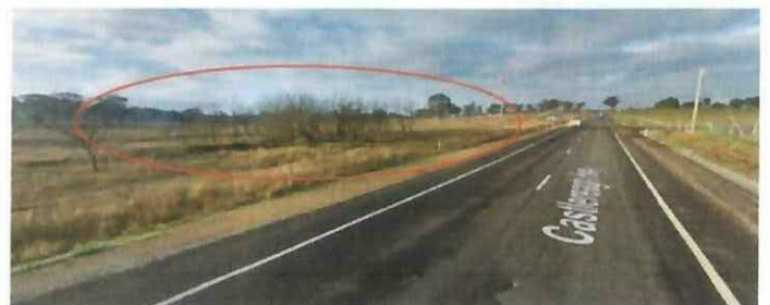
Looking south along Castlereagh Highway toward the site
