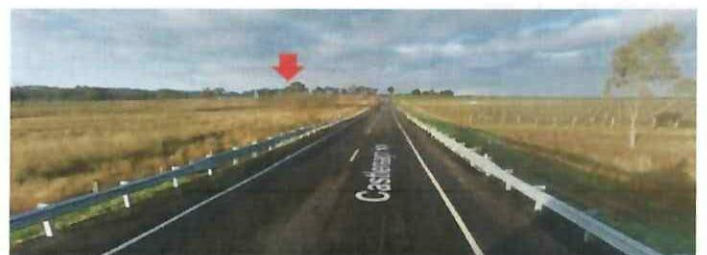
Looking south along Castlereagh Highway toward the site
