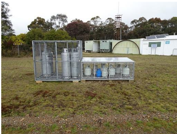
Figure 4-7 – Gas cylinder cages
