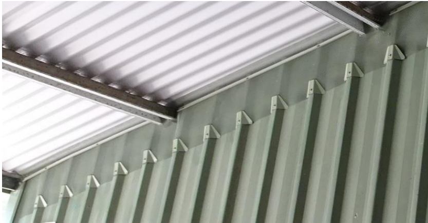
Figure 4-5 – Sealing of internal wall-roof boundary along gable
