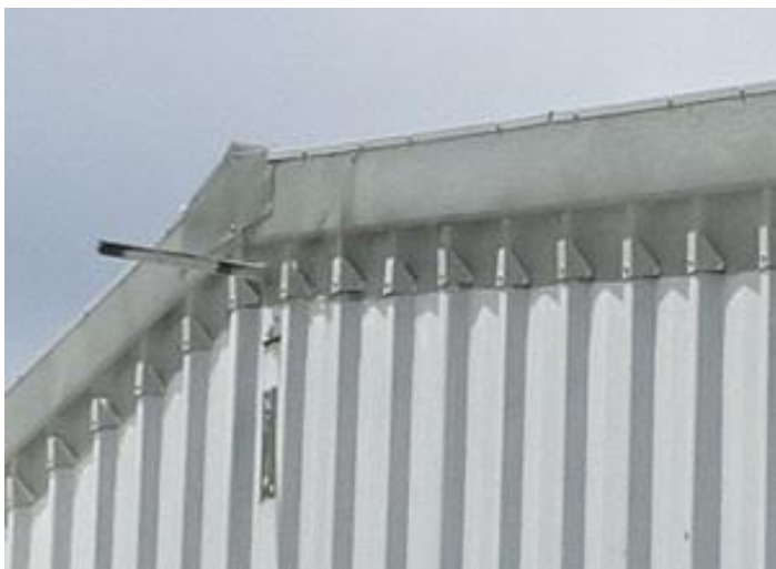
Figure 4-6 – Sealing of external wall-roof boundary on gable
