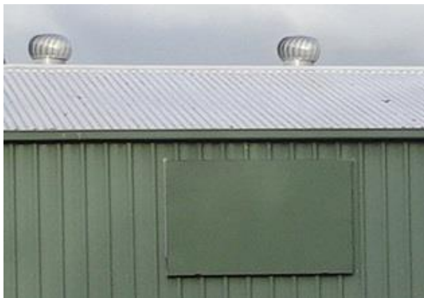
Figure 4-3 – Ember-proofing of roof ridge and windows
