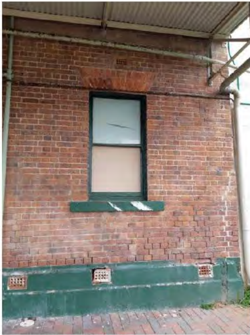
Figure 4.29 | Lewis Street window at NE corner to be refurbished to original state. Brickwork to be re-pointed.
