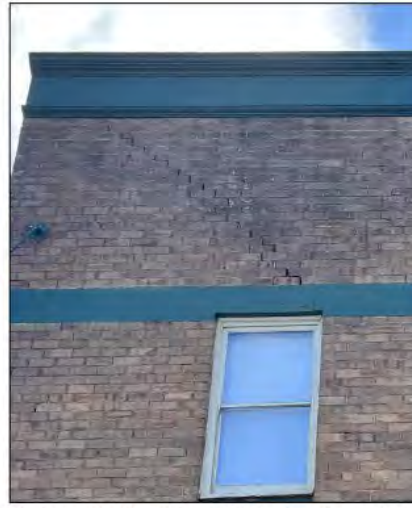
Photograph 10: Federal Hotel external cracking to brickwork at Inglis Street.
