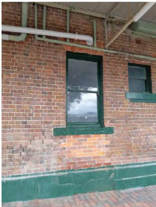
Figure 4.27 | Lewis Street original doorway that has been bricked up. Brickwork to be re-pointed.
