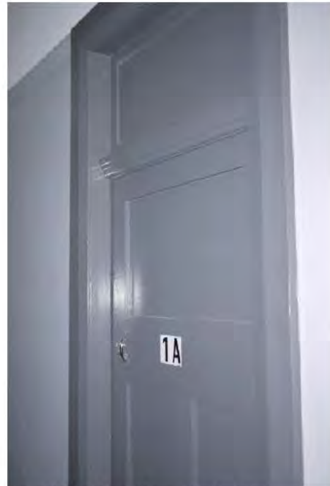
Figure 4.153 | Door of Room 1A showing door frame, transom window and profile of door.
