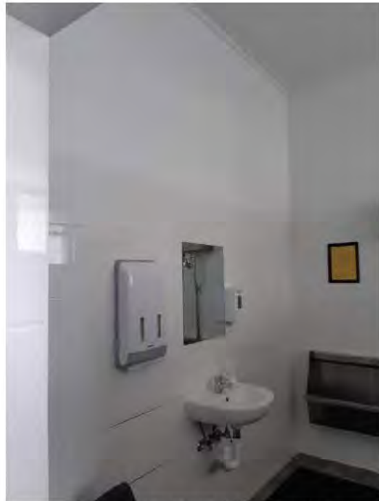
Figure 4.121 | Mens WC in NE wing. To be demolished including internal walls. Nib walls to be kept at external walls.
