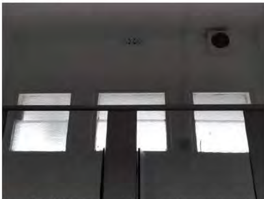
Figure 4.124 | WC windows to be removed and made good. Central window to be re-instated as the originbal timber framed double-hung sash.
