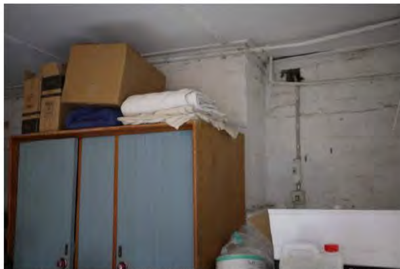
Figure 4.140 | Inside early laundry/kitchen lean-to in NW wing, looking N. Chimney breast behind cupboard to be demolished. Wall at right to be partially retained.
