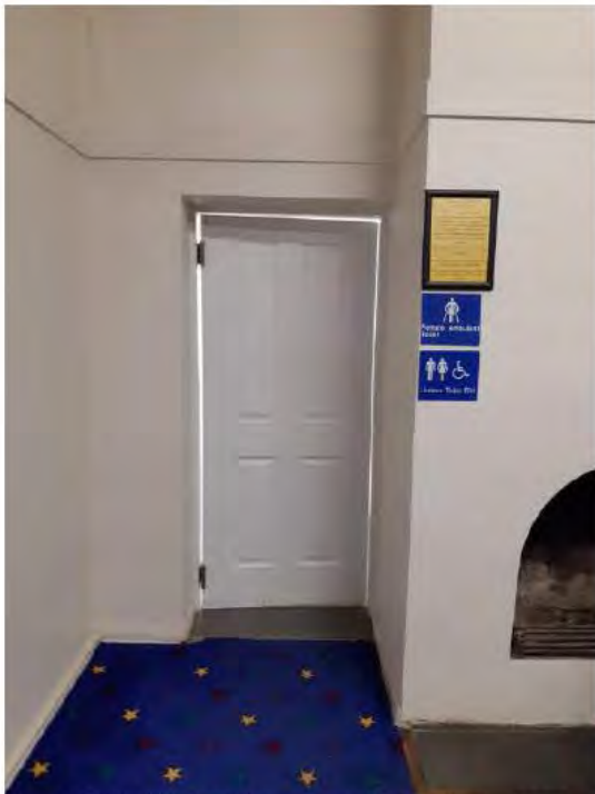
Figure 4.93 | NW wing WCs. Door and left part of wall to be removed for wider access to new WC fitout.
