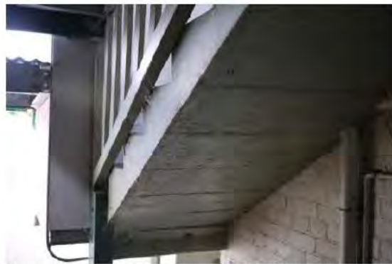
Figure 4.62 | Underside of concrete stairs from former WC on verandah to the mezzanine addition. To be demolished and stair void replaced with decking to match.
