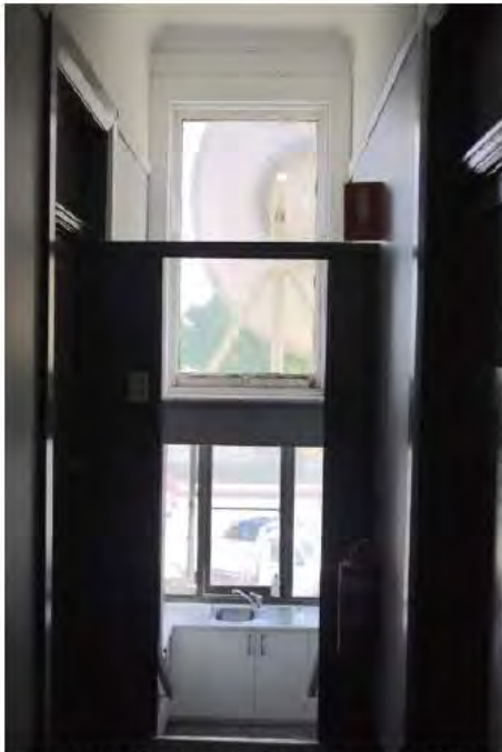
Figure 4.188 | Looking N at the connection of the NE wing of hotel to the 1930s WC mezzanine addition. A doorway will be retained here and connected to a steel walkway from new stairs and lift in the bistro addition.
