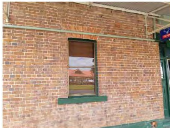
Figure 4.15 | Inglis Street, window to now-gaming room. To be replaced with timber-framed double-hung sash window.
