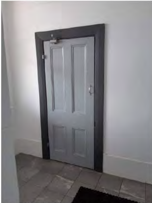
Figure 4.126 | Wall and door to bar area to be removed. 300 mm nib wall to be retained at left.
