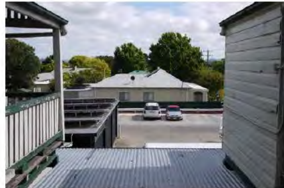
Figure 4.64 | Looking N from rear verandah to the carpark. The corrugated metal roof over the ground courtyard is to be removed. A double storey glazed wall will be erected across the end of the hotel and courtyard between the old, and the new bistro addition.
