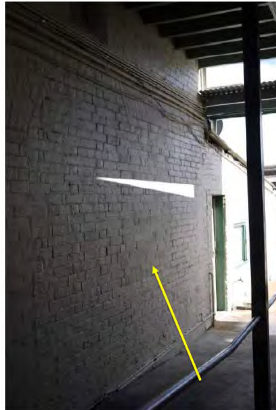
Figure 4.39 | E wall of the NW wing. Bricked-up original window. Paint to be removed from brick.
