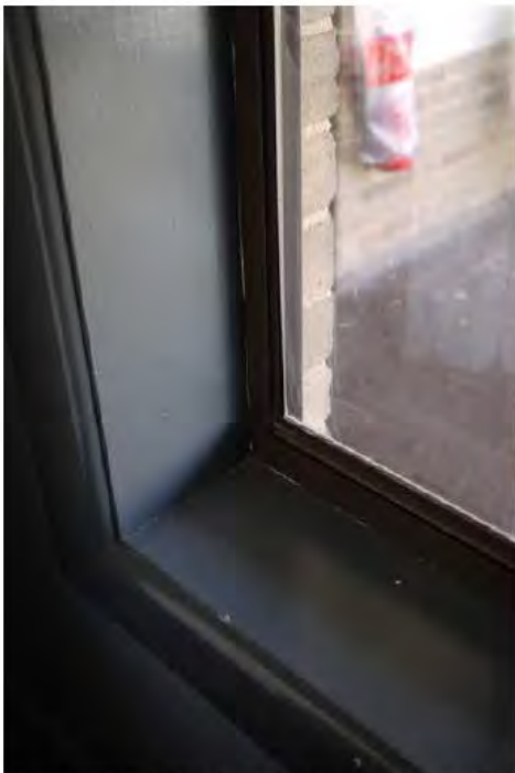
Figure 4.184 | Original timber window sill and architraves.
