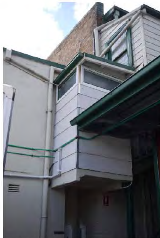
Figure 4.57 | View E looking at the Lewis Street 1930s mezzanine addition, which is to be removed, along with the stairs to it from the first floor verandah.
