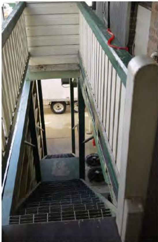
Figure 4.60 | Modern steel staircase to be removed and decking replaced over the void in the verandah.
