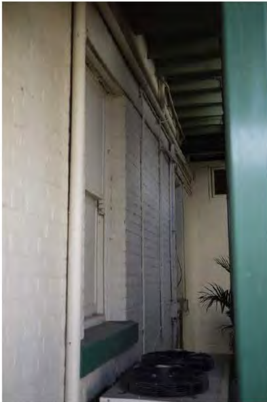
Figure 4.33 | Looking S at W side of the Lewis St wing. Paint to be removed to expose face brick. Windows to be refurbished to original state.
