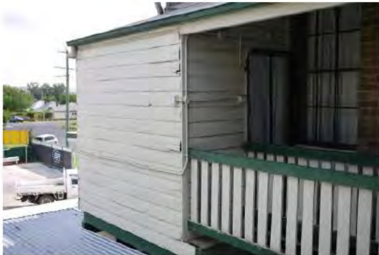
Figure 4.58 | Former WC on the NE corner verandah. Enclosure to be removed and reconstructed to match rest of verandah form and detailing.
