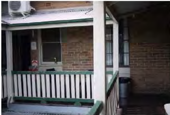
Figure 4.63 | Rear of Inglis Street frontage. Aluminium window at right to be replaced with a timber framed double-hung sash window like the one at left.
