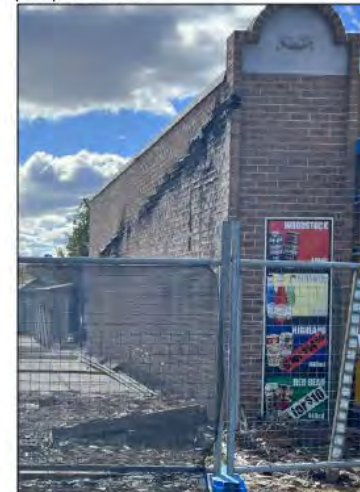
Photograph 13: Federal Hotel bottle shop wall damage by fire at 38 Inglis Street.
