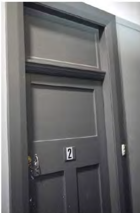
Figure 4.154 | Original door and frame to Room 2. Appears transom glazing has been retained and painted over.
