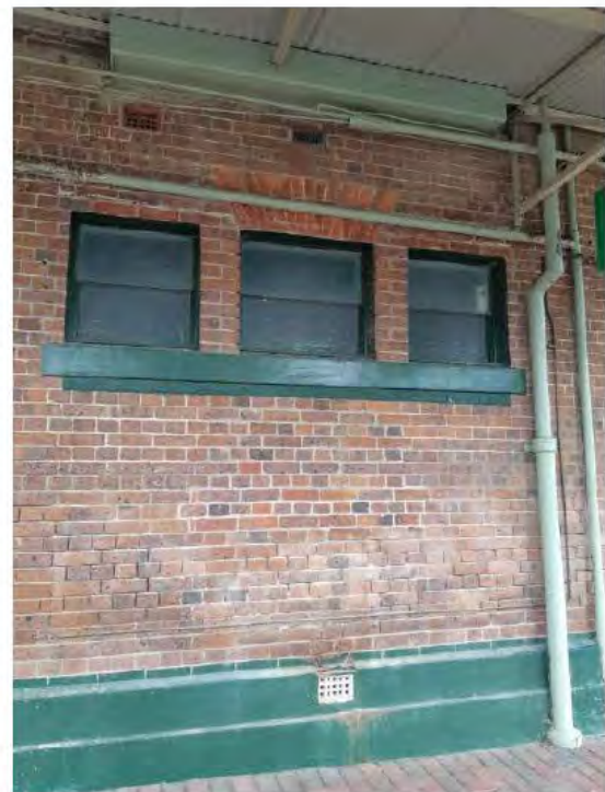
Figure 4.28 | Mid-century WCs alteration removed an original window; header still evident. Remove 3 x high windows and sill. Reconstruct central timber-framed double-hung sash window and sill to match existing. Bricks to be re-pointed.
