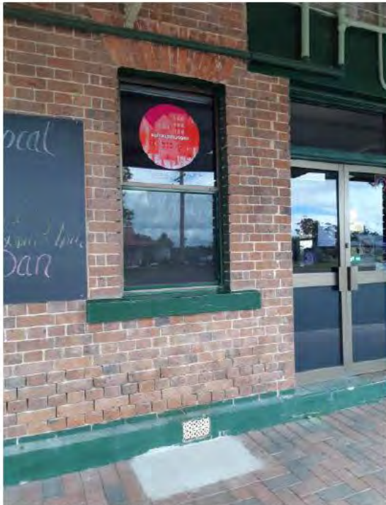
Figure 4.21 | Inglis St public bar window and door. To be replaced by era-appropriate timber framed windows and doors. Brickwork at base of wall to be re-pointed.
