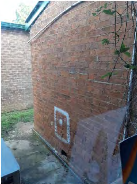
Figure 4.47 | S end of the NW storeroom. Walls to be partially retained and incorporated into new design. This window to be altered into a doorway.
