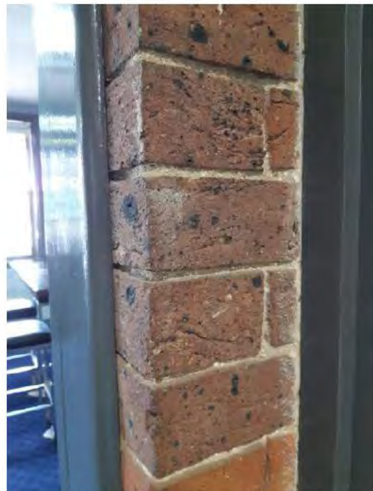
Figure 4.133 | Detail of 1880s sandstock brick at right of doorway.
