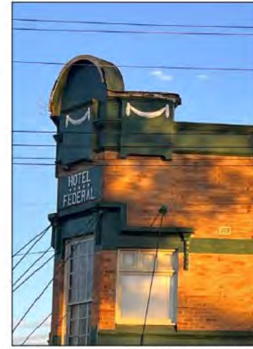
Photograph 10: Federal Hotel deterioration of parapet details.
