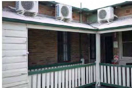
Figure 4.61 | Intersecting corner with the Inglis St frontage. Windows at left to be replaced with windows like that at right.
