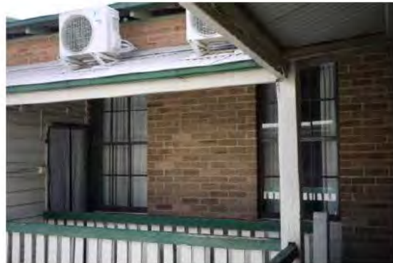
Figure 4.59 | NE wing windows to be reconstructed to timber-framed double-hung sash windows.
