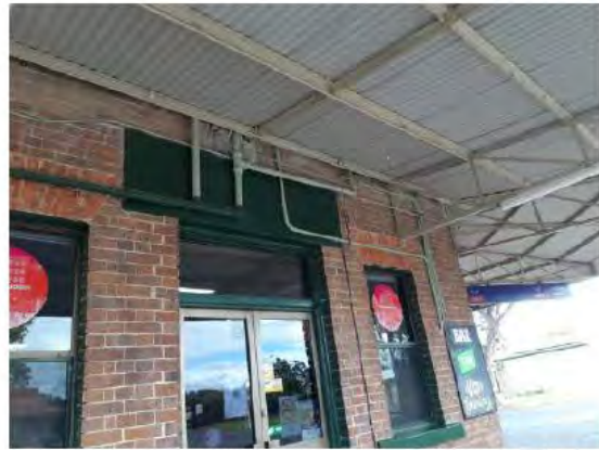
Figure 4.22 | Doors and window to be replaced with timber-framed era-appropriate doors and windows.
