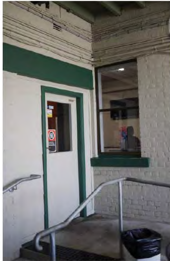
Figure 4.37 | Rear courtyard. Door to Inglis Street entrance hallway at left. Aluminium window frame to be replaced with timber-framed double-hung sash.
