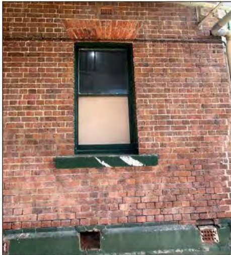
Photograph 9: The Federal Hotel deterioration of external brickwork as viewed from Lewis Street.
