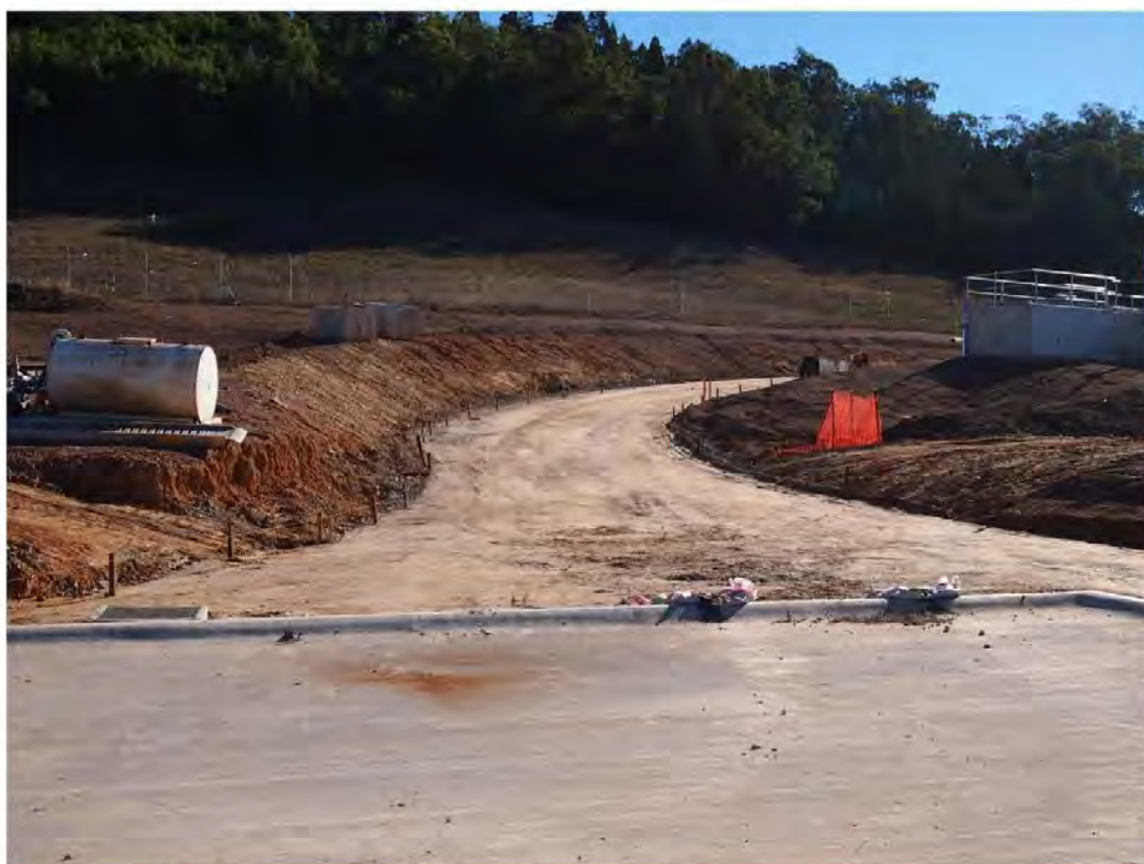
Photograph 1. Roadworks prior to kerb construction
