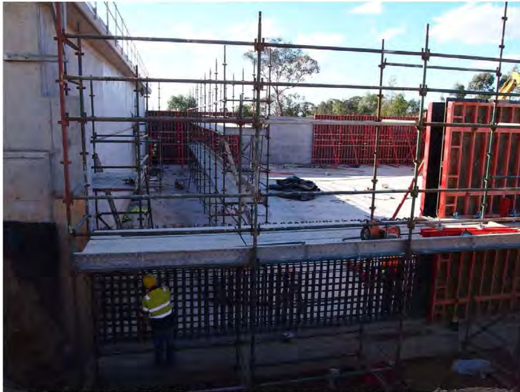
Photograph 2. Re-construction of final section of balance tank wall.
