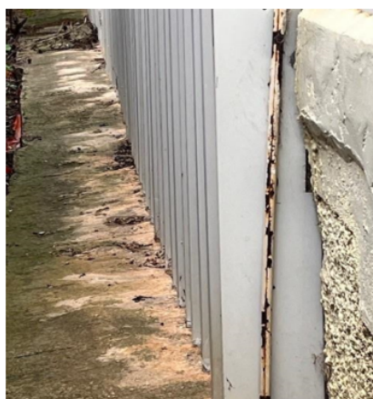
Figure 6 front LH corner showing the end of ground retaining beam or shoring.
