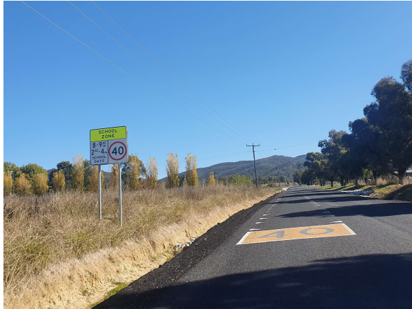
Open stormwater channel leaves no space to walk away from traffic.
