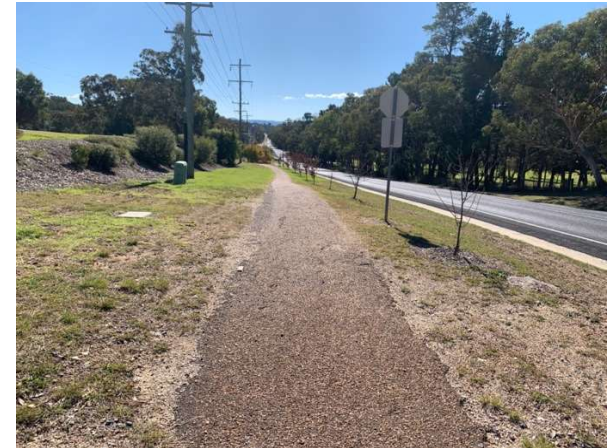
Uneven, narrow, unshaded and unsigned bike track between Kandos and Rylstone.
