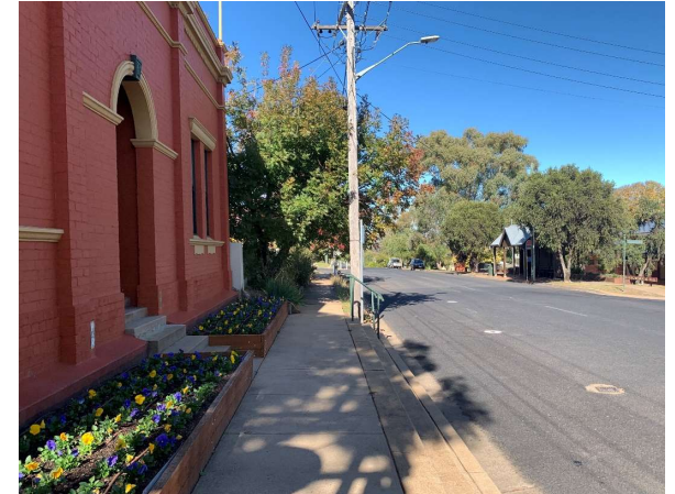
The footpath outside the museum in Gulgong is narrow and has high steps, limiting accessibility.
