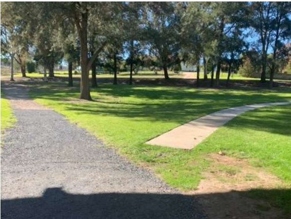
Missing connection from the gravel shared path to a footpath near the Cudgegong River.
