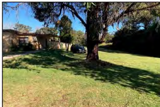
Figure 20. External view of the garden space on the eastern side of the subject residence. Taken from the south side of Horatio Street, facing south.
