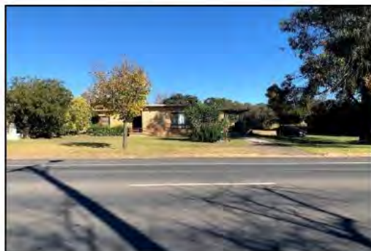
Figure 18. External view of the primary (northern) façade of the dwelling on the subject site (Post-War residence). Taken facing south from the north side of Horatio Street.
