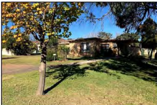
Figure 19. External view of the primary façade of the dwelling on the subject site. Taken from the southern side of Horatio Street, facing south-east.
