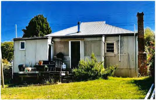
Figure 4: Figure 5 Rear view of residence showing hipped roof and chimney that will be retained. The small rear verandah , partially enclosed, and rear linings and wall will be removed. Image 13 December 22.
