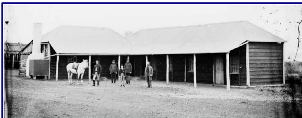
Figure 4 - Gulgong Police Station, Barracks and Lockup (circa 1870 – 1875)
