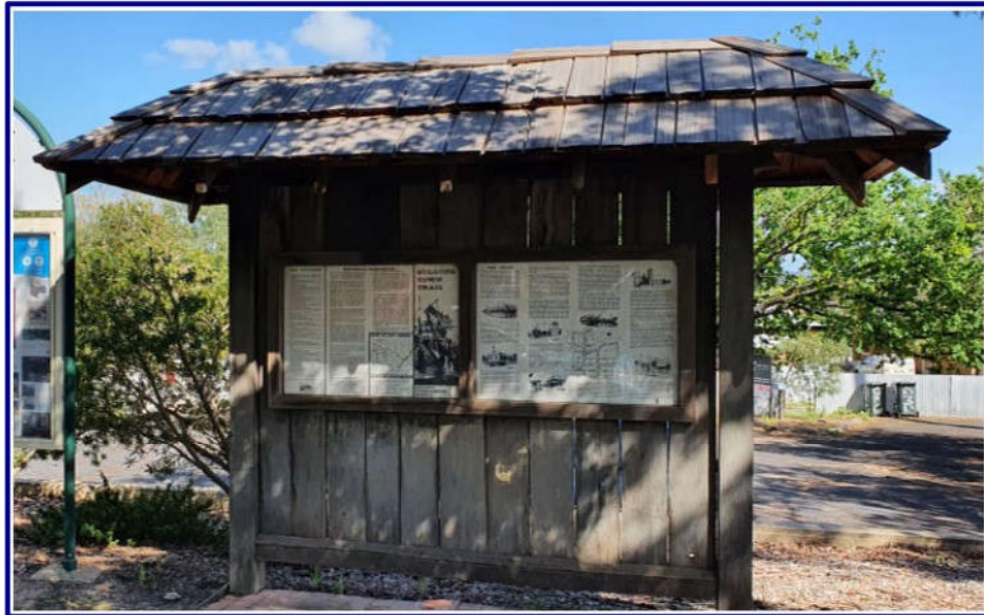
Figure 9 - Gulgong Town Trail shelter
