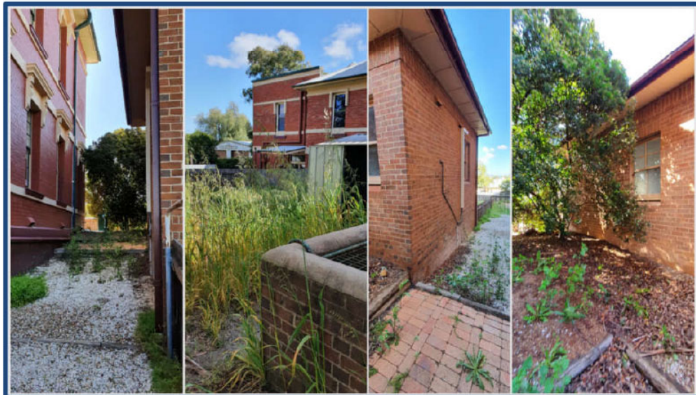
Figure 15 - Fire Station Side Boundaries (L-R) Beyond northern boundary adjoining property (adjoining property), view across back to adjoining property, northern wall facing west and northern wall facing east.
