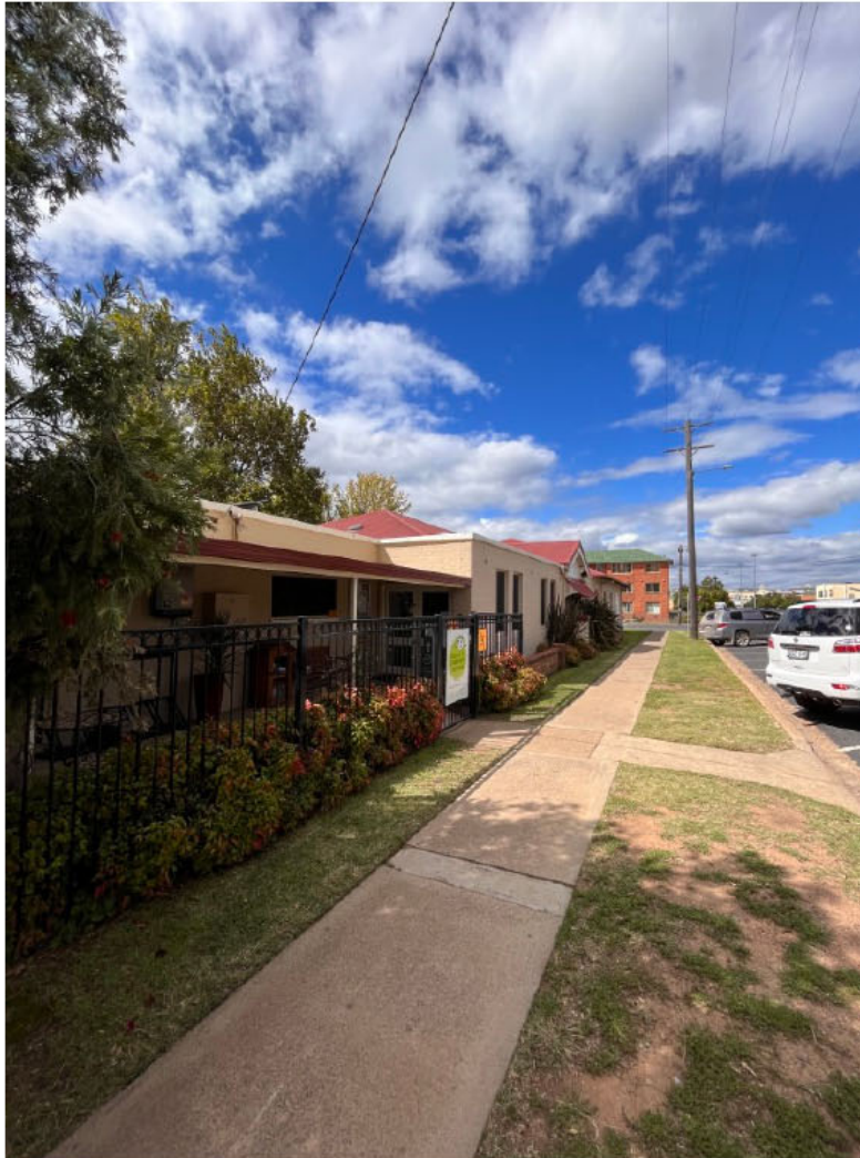
Figure 2: Photo of existing kerb ramp on Lovejoy Street
