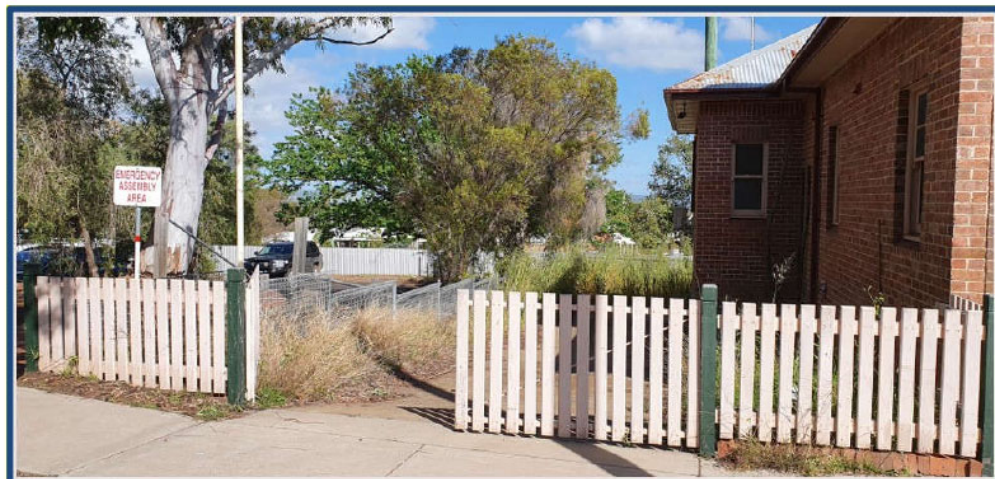
Figure 19 - Fire Station External Assets Fire Station picket fence on Herbert Street boundary, and boundary of adjoining car park to the south showing ringlock fencing. (Note mature Eucalypt tree near car park)
