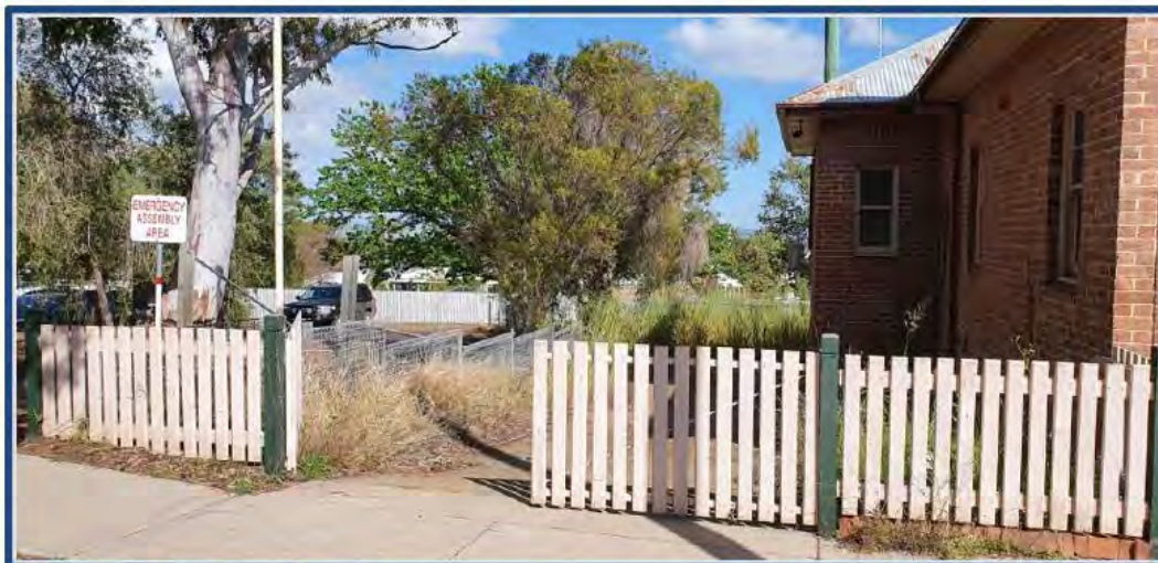
Figure 19 - Fire Station External Assets Fire Station picket fence on Herbert Street boundary, and boundary of adjoining car park to the south showing ringlock fencing. (Note mature Eucalypt tree near car park)
