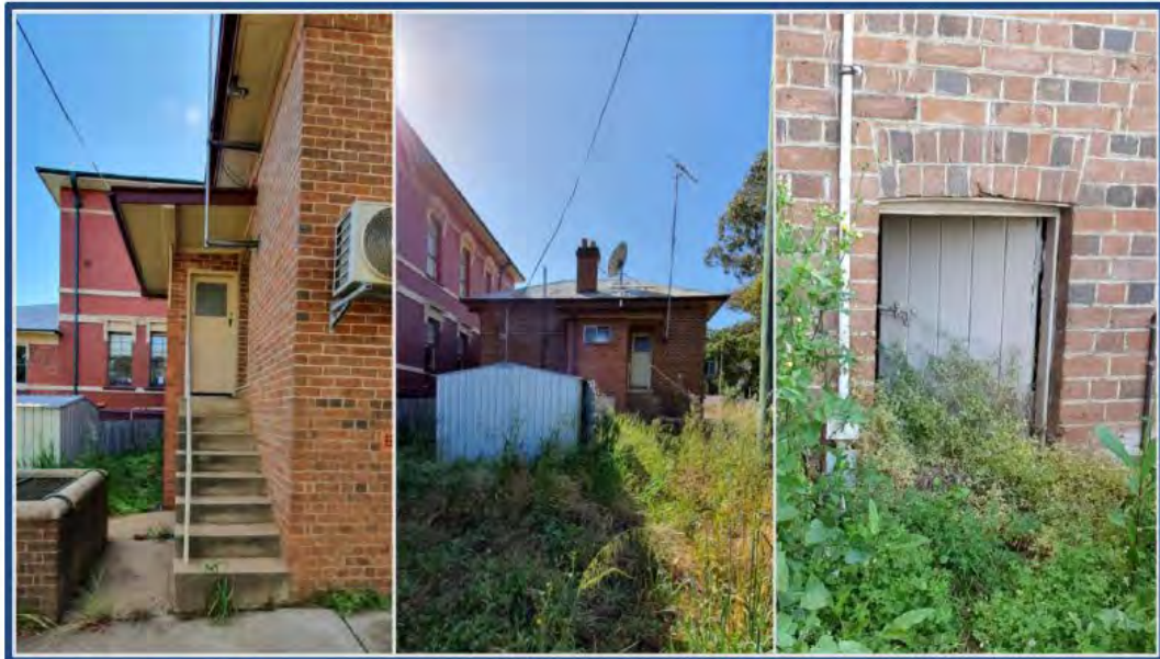
Figure 14 - Fire Station Rear (L-R) Rear entrance, rear view with garden shed, access to subfloor storage area.
