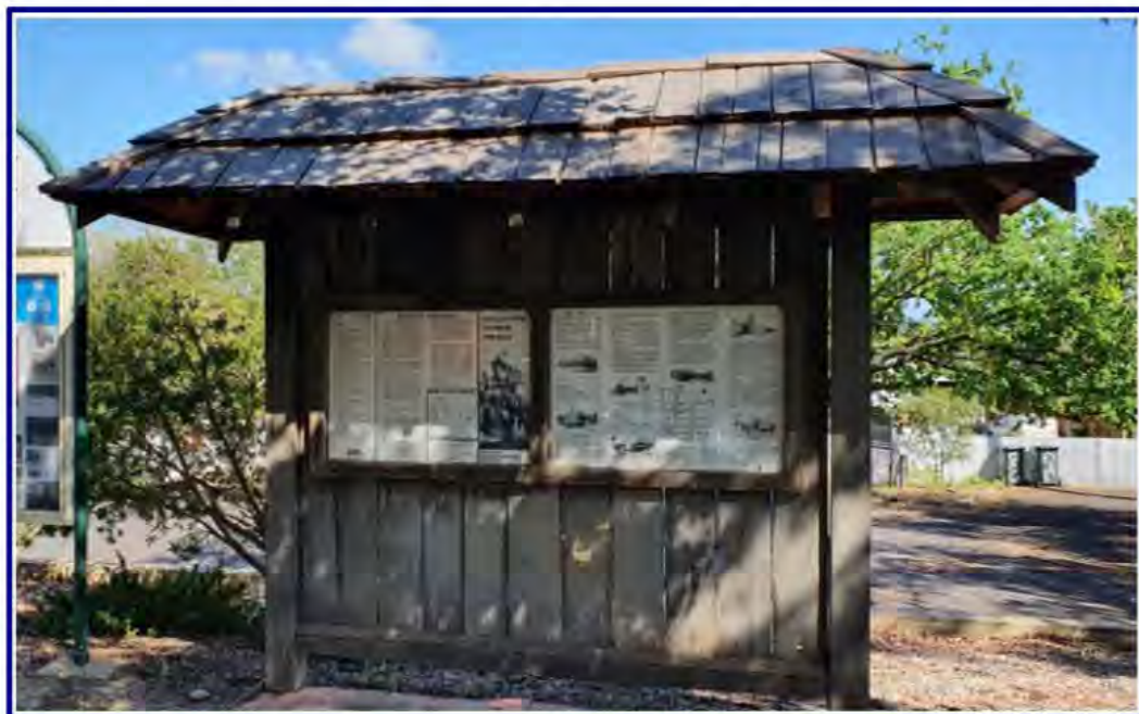
Figure 9 - Gulgong Town Trail shelter
