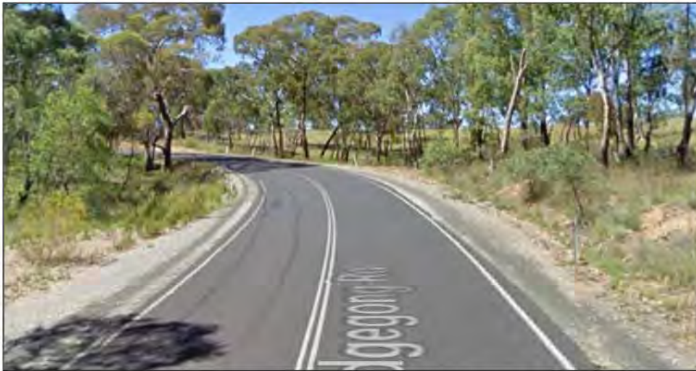
FIGURE 3.1 TYPICAL VIEW OF CUDGEGONG ROAD
