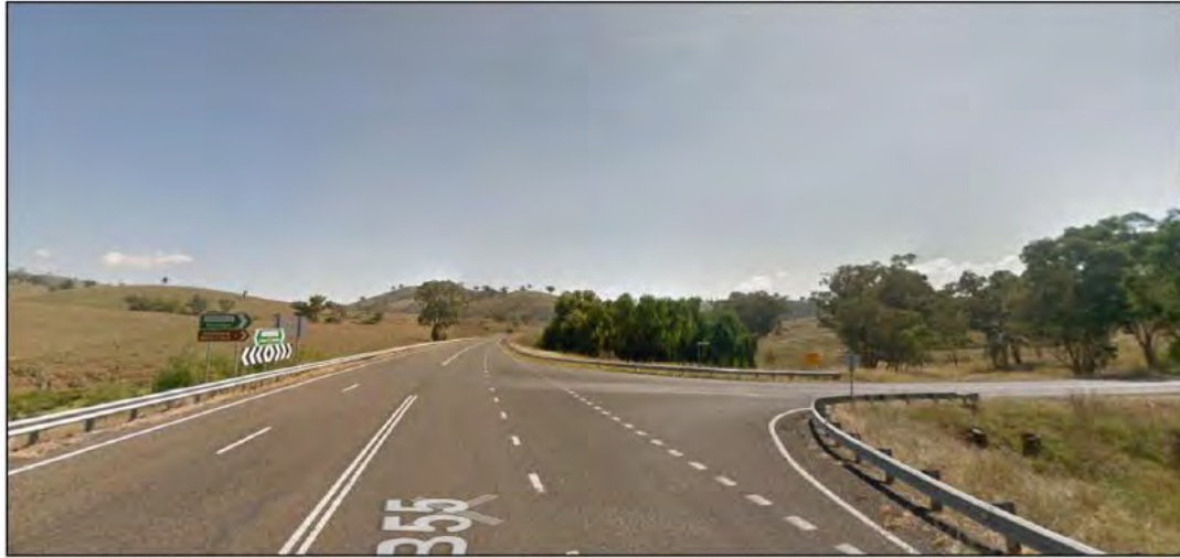
FIGURE 3.2 CUDGEGONG ROAD / CASTLEREAGH HIGHWAY INTERSECTION
