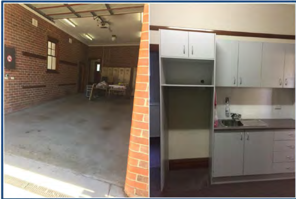
Figure 12 - Fire Station Internal Garage (left) and kitchen.
