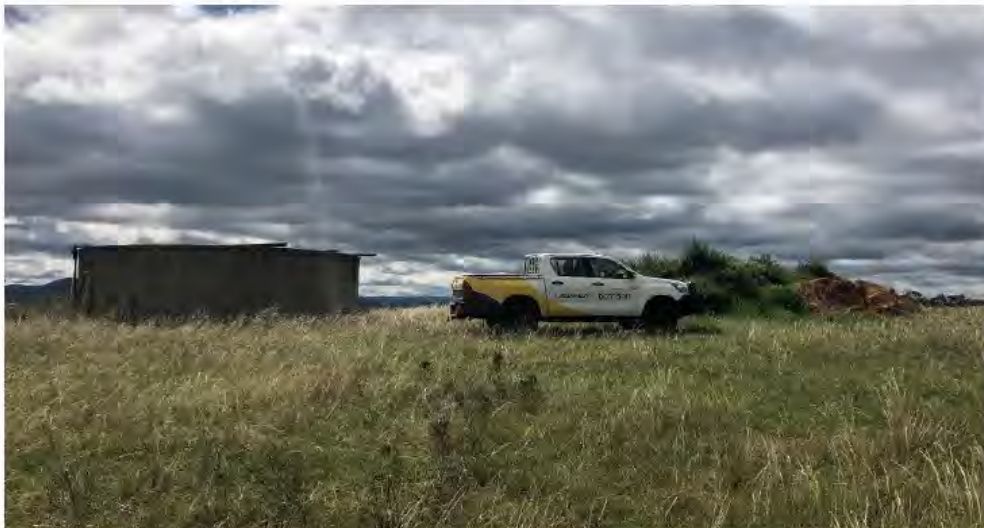
Figure 6.6: Concrete dam and fill stockpile at the top of the rocky outcrop.
