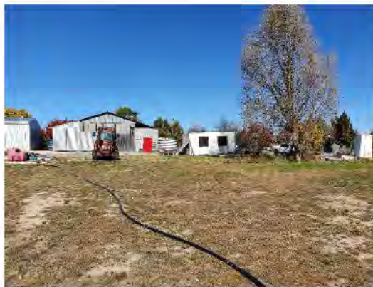
Plate 2.6 View west showing farm shed and other outbuildings associated with the commercial winery
