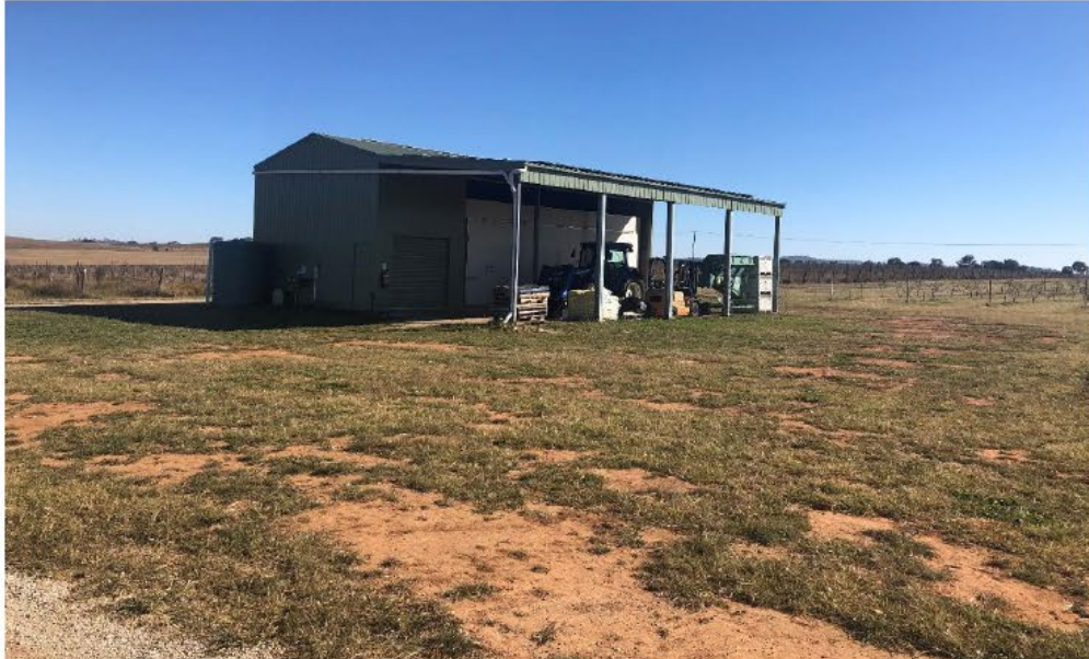
Figure 2.4: Picture from point C, showing packing shed.
