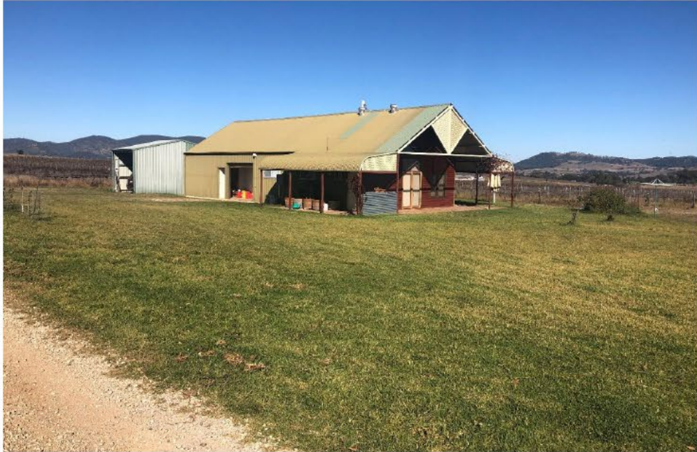
Figure 2.6: Picture from point E, showing cottage and attached equipment storage shed.
