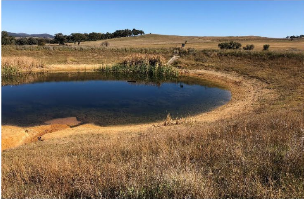
Figure 2.8: Picture from point G, showing turkeys nest dam.
