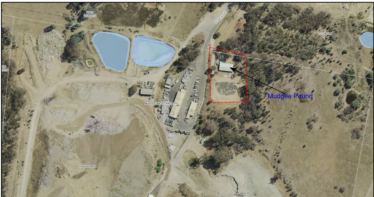
Figure 1 - Aerial image of existing pound and surrounds (Source: Extract from plans provided with the application)
