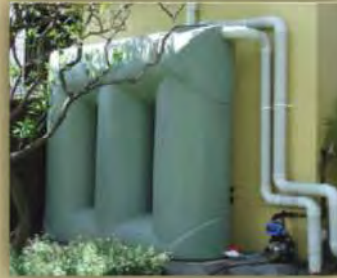
Rainwater tanks collect water which can be used for irrigation or for toilet flushing, etc, which helps to minimise our use of potable water.
