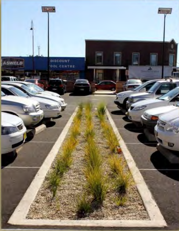
Raingardens filter pollutants off impermeable surfaces, such as car parks, and add amenity to public spaces.
