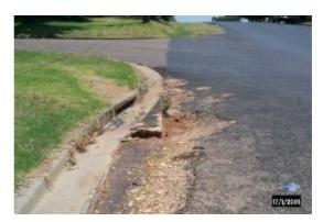
**Photo 7.** Insufficient road maintenance can lead to roadside erosion, as seen here in Gulgong
