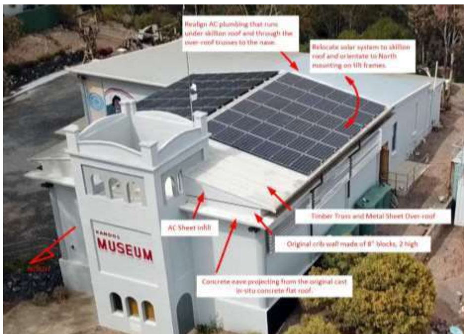
Figure12: Aerial view of Kandos Museum illustrating works to be undertaken to reveal Floyd's Roof. Photo credit Kandos Museum 2019.
