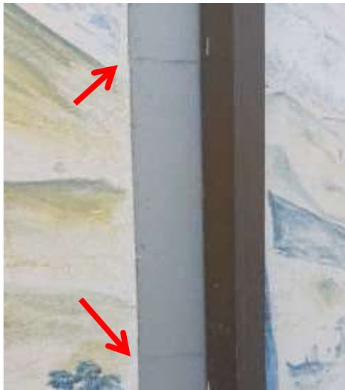
Figure 10: Section of one of the "8 poles" of the nave constructed on-site using slip-form technique showing witness marks to successive pours to form a column of 16" (400mm) diameter. Photo credit Kandos Museum 2022.
