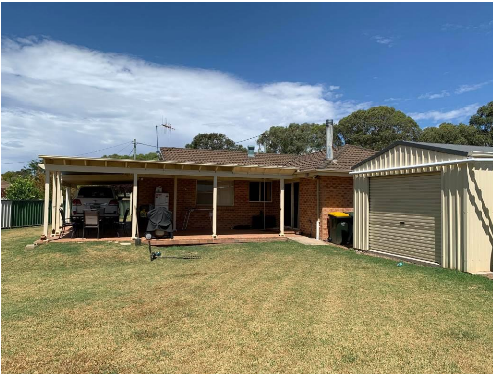
Plate 1 – South facing view.
