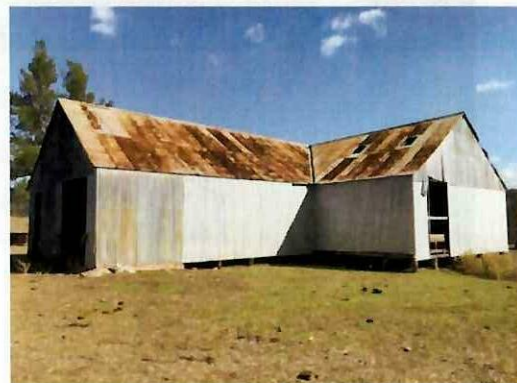
Figure 5 Former Shearing Shed
