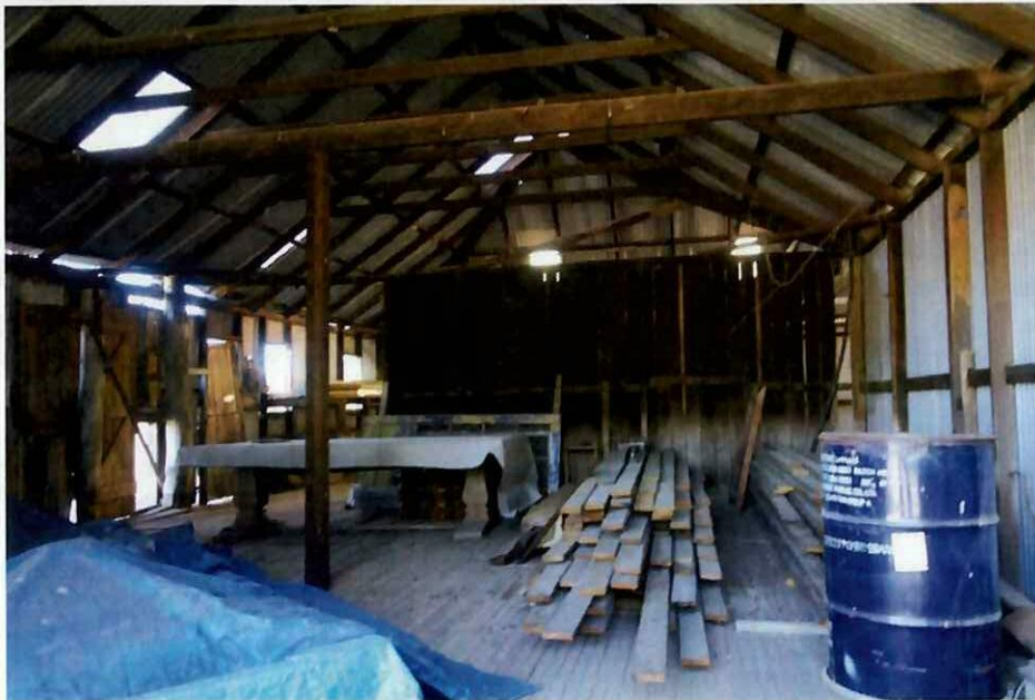
Figure 3 interior view of shearing shed.
