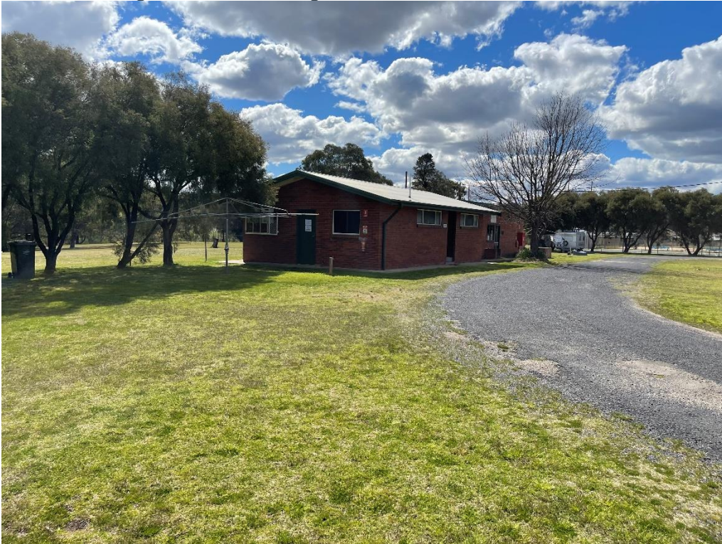
Photo 5: Existing amenities building
