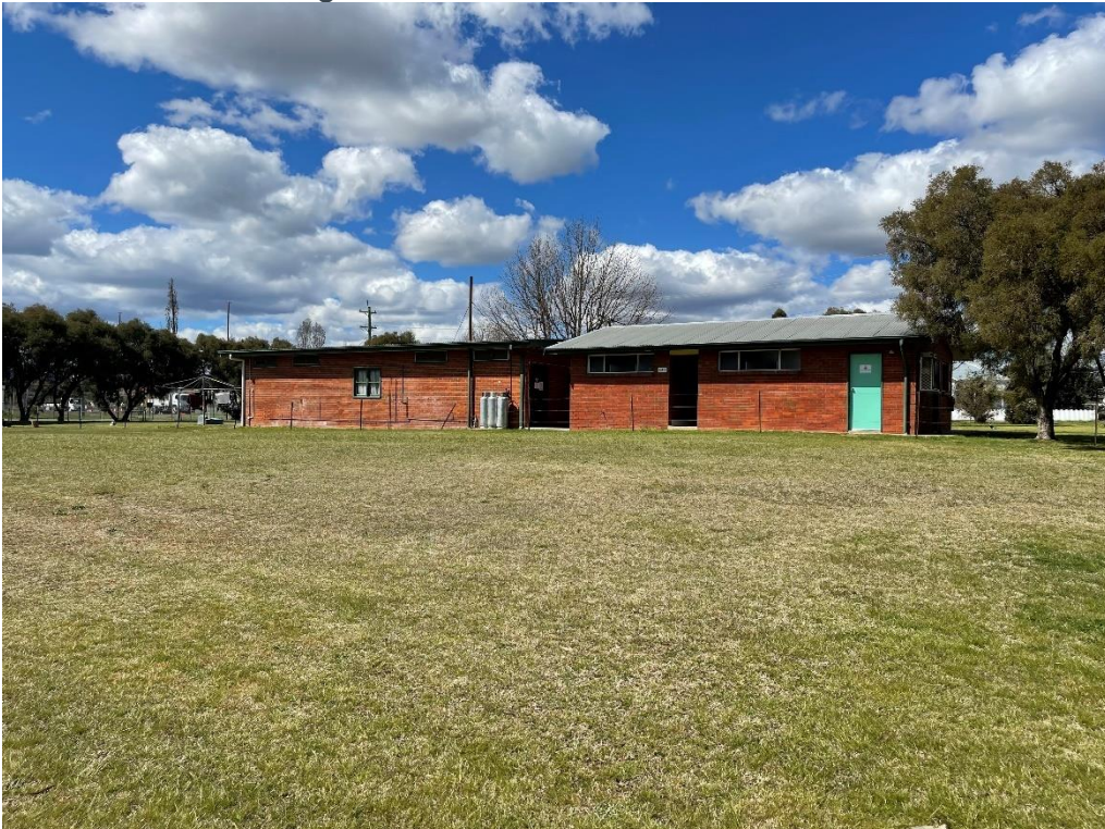
Photo 4: Rear of existing amenities
