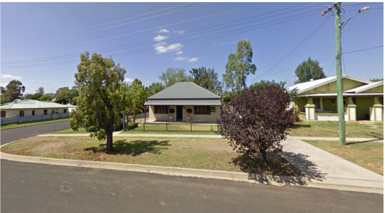
Plate 1 – View of the site fronting Gladstone Street (Google Street View)
