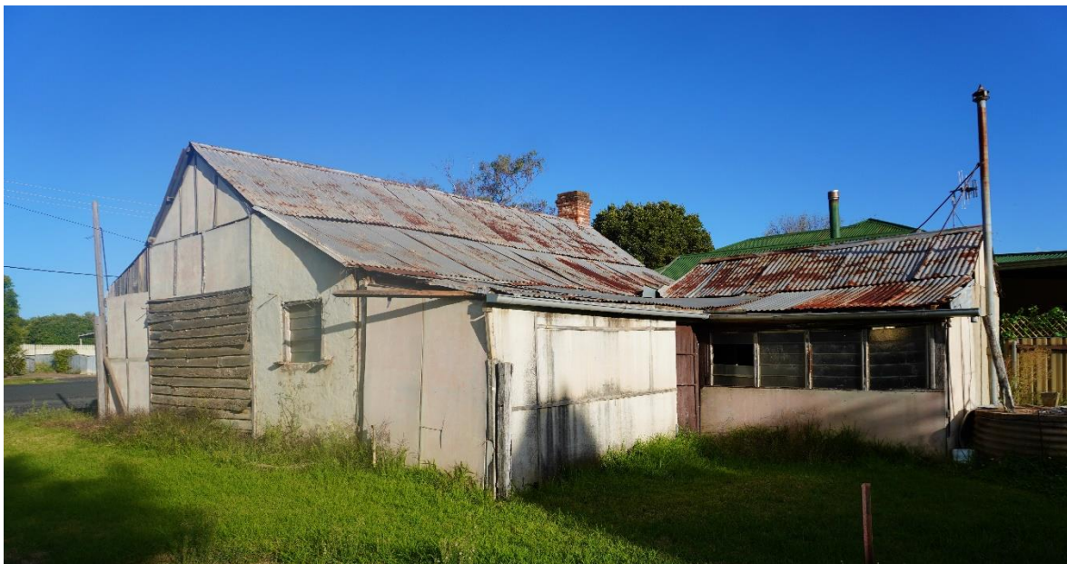
FIGURE 5 VIEW FROM THE NORTH SIDE
