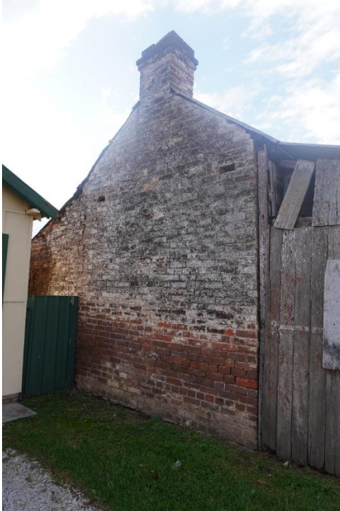
FIGURE 6 SOUTH FACING GABLE SHOWING THE ORIGINAL ENGLISH BOND BRICKWORK.
