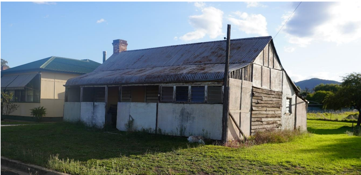
FIGURE 1 FAÇADE OF EXISTING HOUSE AT 66 COX STREET MUDGEE
