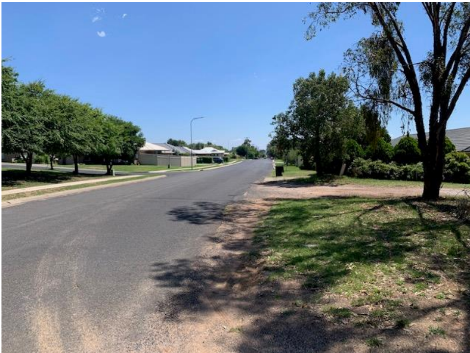
Plate 3 – View of Robertson Street and access to the existing dwelling
