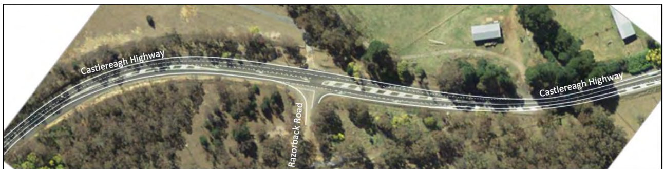
Figure 11: Intersection of Razorback Road and Castlereagh Highway
