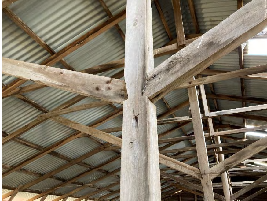
Plate 6 Mortise join on centre post uprights are a feature of the construction. Photo: Darrell Rigby 19.5.2022.
