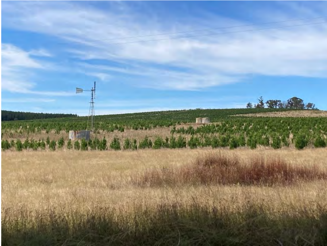
Plate 12 Concrete water tanks and windmill infrastructure. Photo: Darrell Rigby 19.5.2022.
