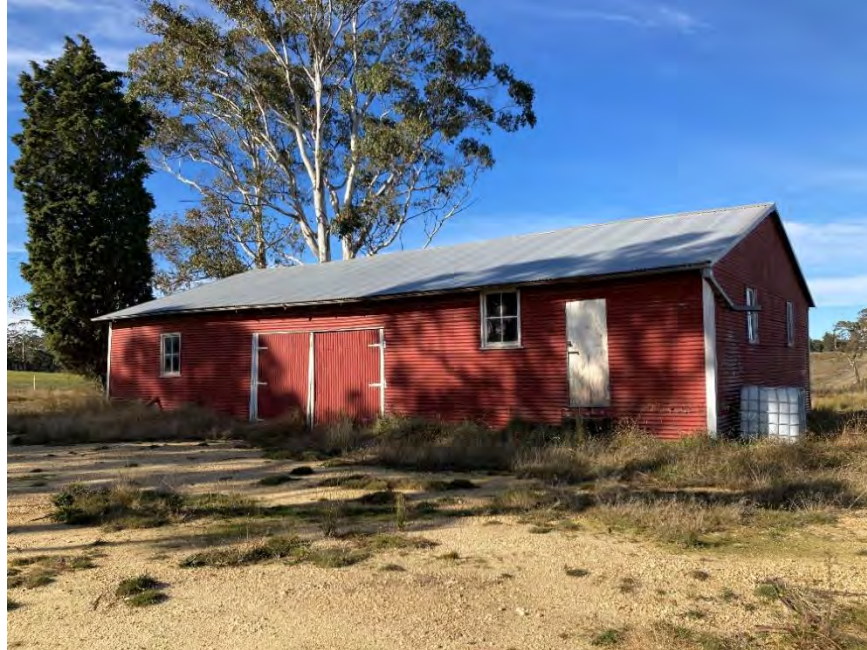
Plate 3 machinery shed northwestern \frac{3}{4} elevation. Photo: Darrell Rigby 19.5.2022.
