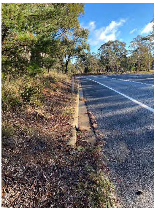
Photograph 11 Embankment to north of Intesection
