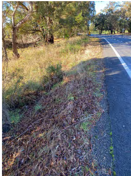
Photograph 8 Embankment inside of curve southbound Castlereagh Highway
