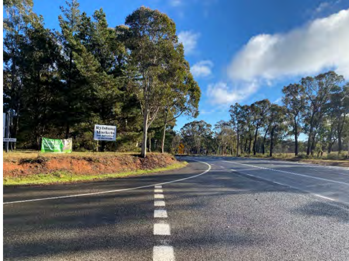
Photograph 9 Embankment to north of Intesection
