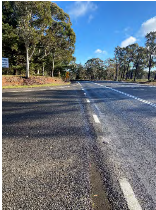
Photograph 10 Embankment to north of Intesection
