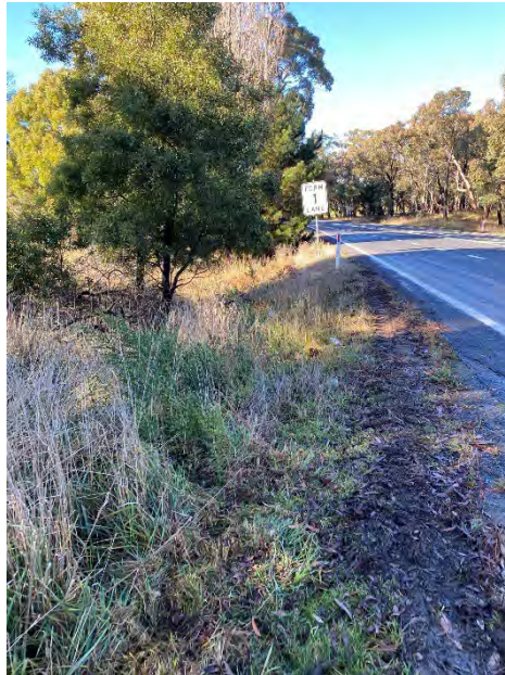
Photograph 7 Embankment inside of curve southbound Castlereagh Highway
