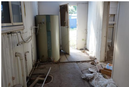
Figure 6 Rear side entry enclosed space with
