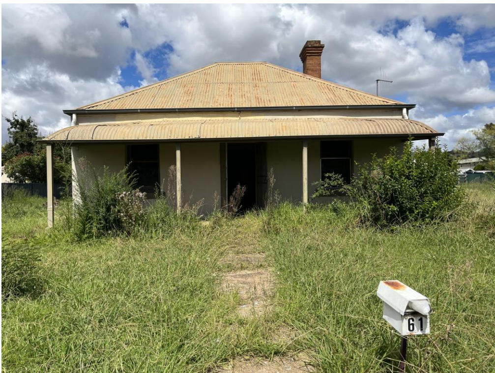
Plate 3 – View of the dwelling to be demolished.
