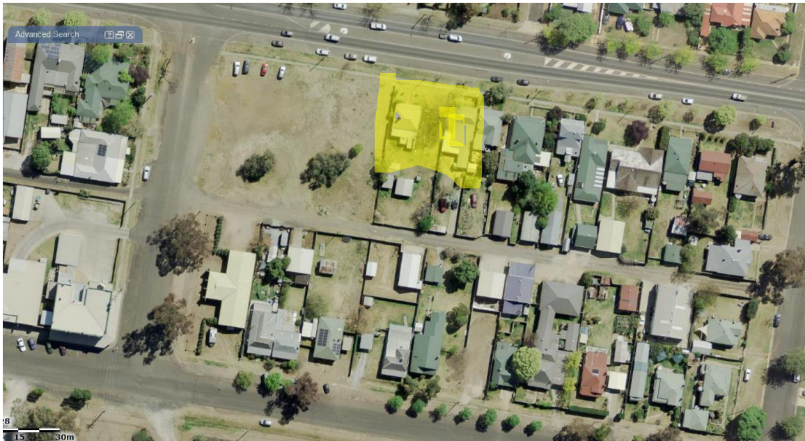
Figure 1: Aerial view of the proposed site for the Motel. Houses at 59 and 61 Horatio Street, to be demolished are highlighted.
