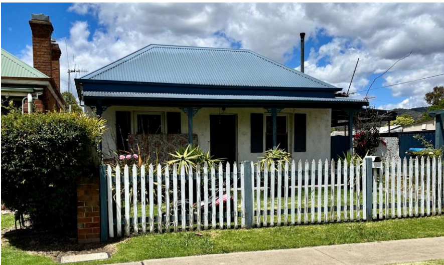
Figure 9 Front view of 59 Horatio Street
