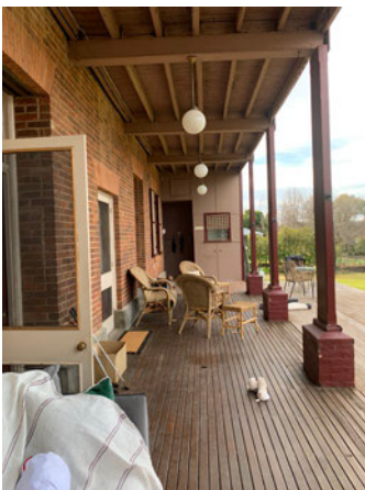
Figure 9: Eastern ground level verandah with enclosure at north-eastern corner.
