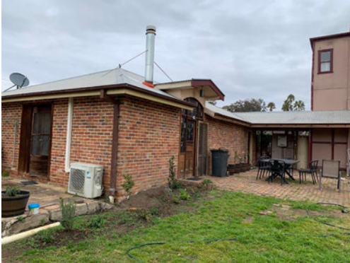
Figure 5: Existing secondary dwelling, to the southeast of the main house.
