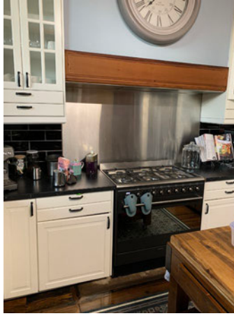
Figure 13: Original chimney breast partially removed by previous owners to accommodate stove. A new door opening is proposed in this location.
