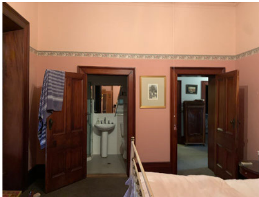
Figure 17: View of later addition door opening into ensuite from Bed 1.
