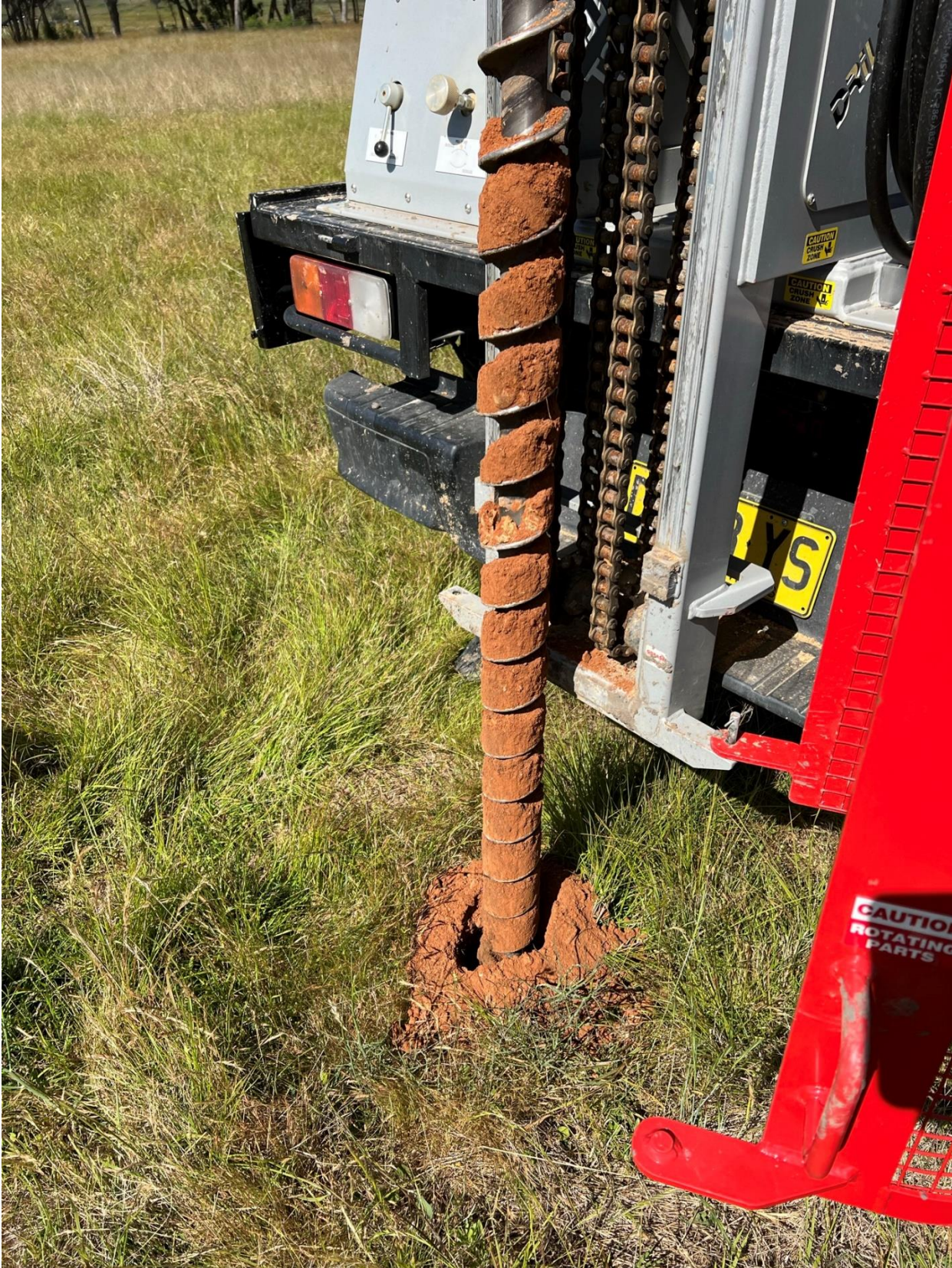
Figure 3: Borehole 1 excavated onsite
