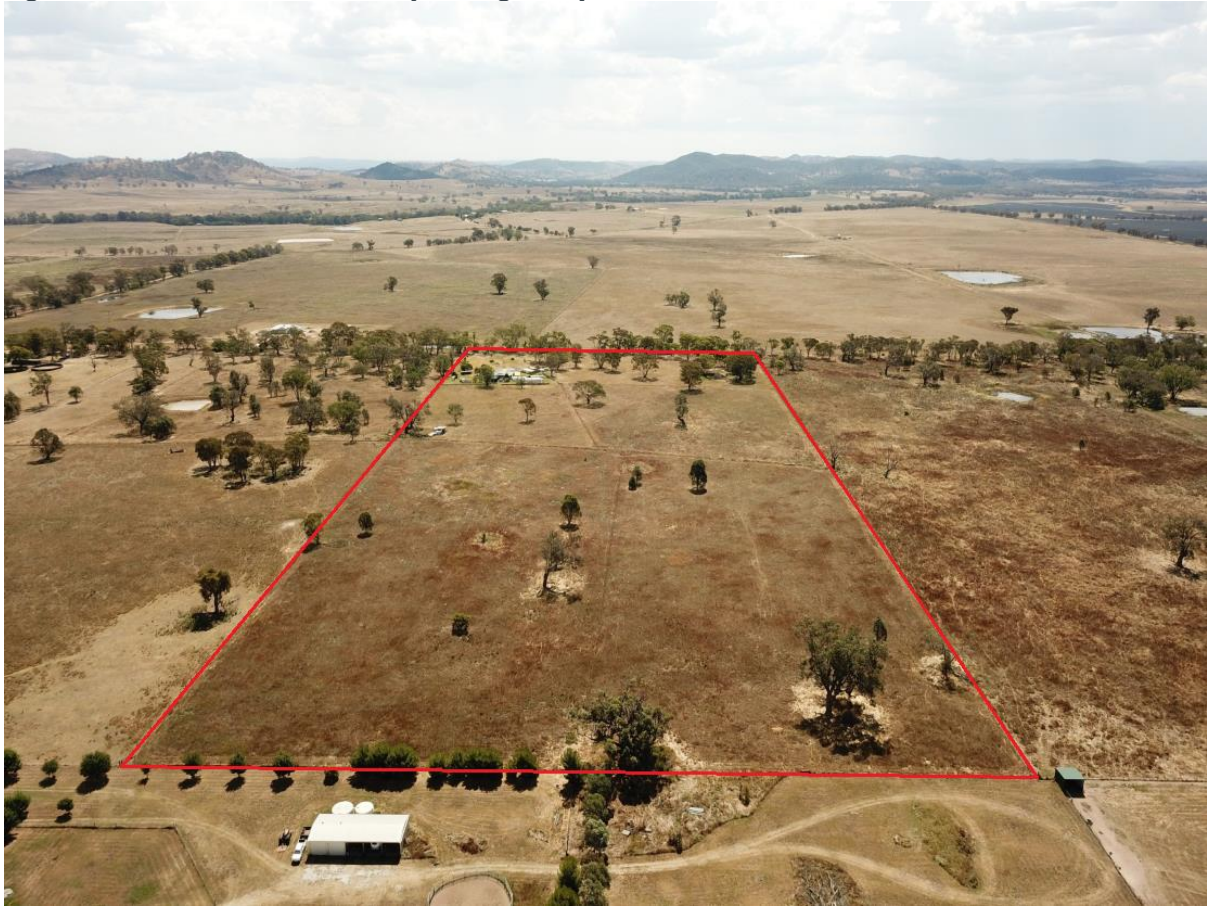
Figure 2: Aerial View of the Site (looking west)
