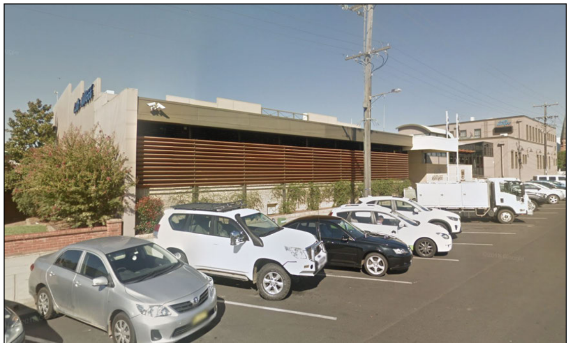
Figure 6: View from Mortimer Street.
