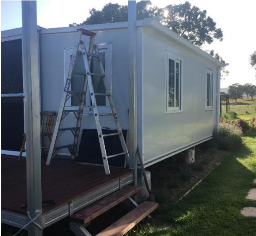
Photo 3: Side (northern) Elevations – Tourist Accommodation Units
