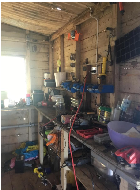
Photo 7: Inside of former post office
