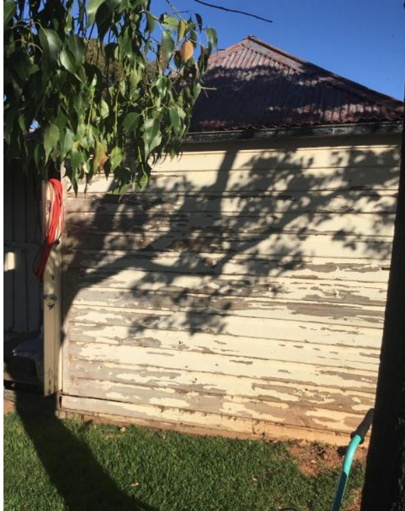
Photo 4: View from west of the building
