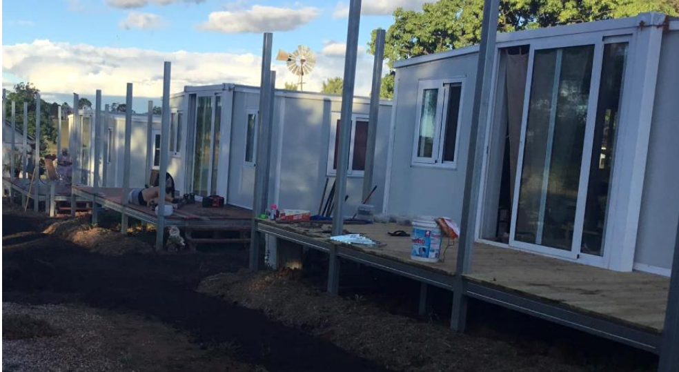
Photo 1: Front Elevations – Tourist Accommodation Units
