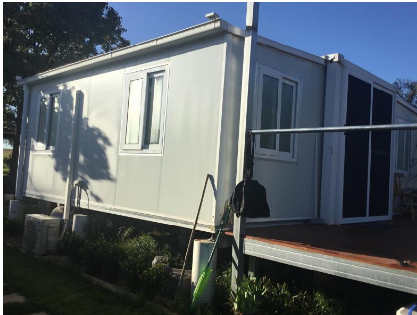
Photo 4: Side (eastern) Elevations – Tourist Accommodation Units
