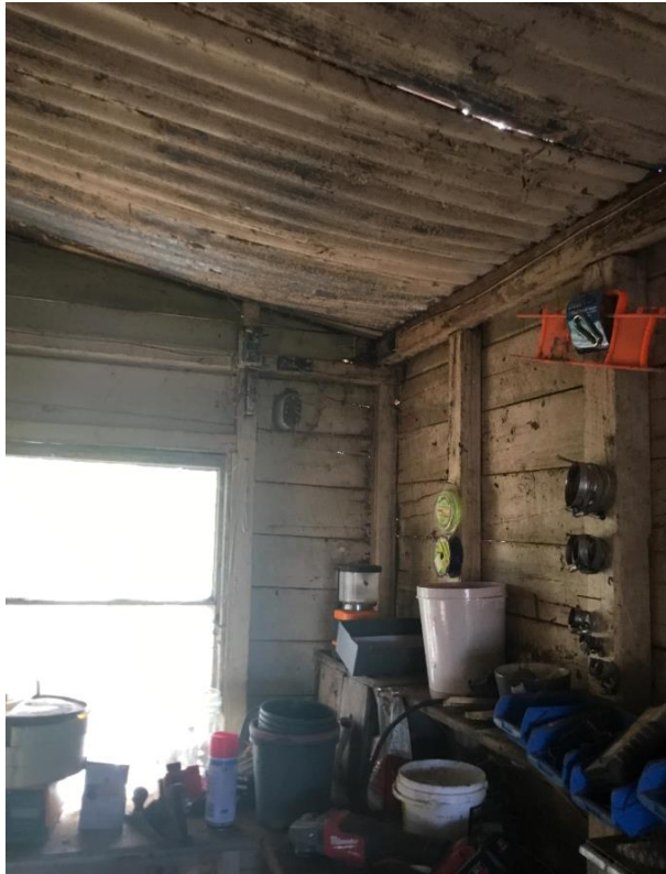
Photo 6: Inside of former post office
