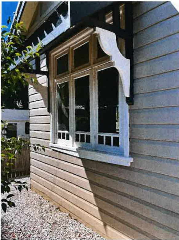
Figure 7 Front window detail
