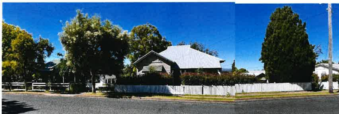
Figure 6 Mayne Street Streetscape
