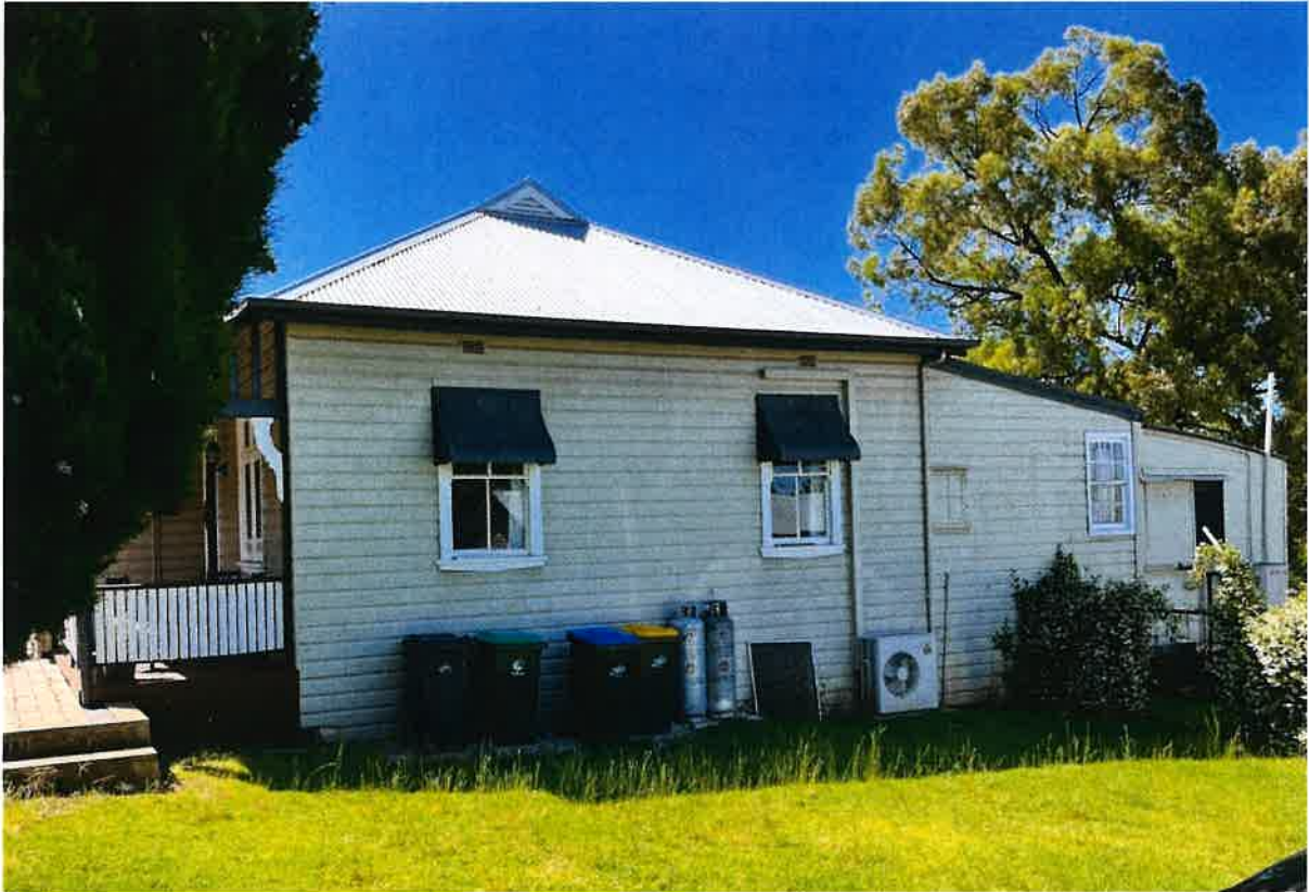
Figure 3 Side view of house at 74 Mayne St. Image 13 December 22
