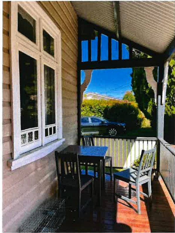
Figure 8 Front verandah detail
